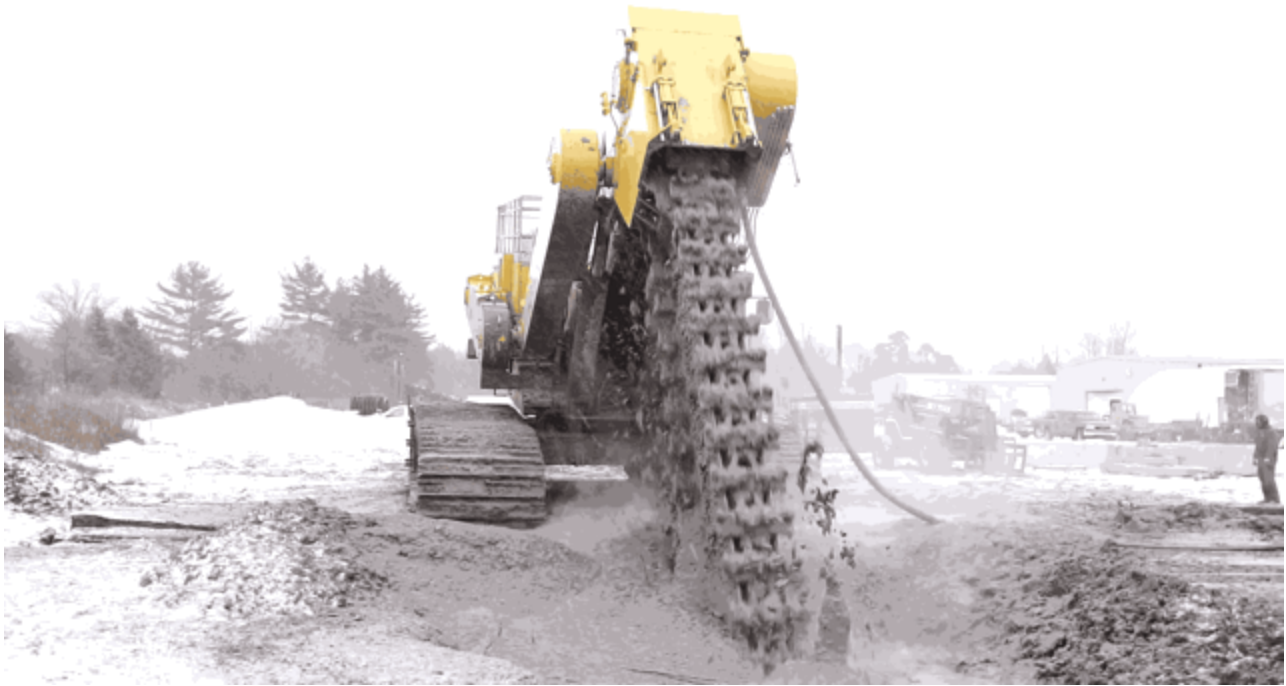
Mix in place walls
