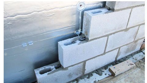
Polyiso wall insulation on a commercial building.
