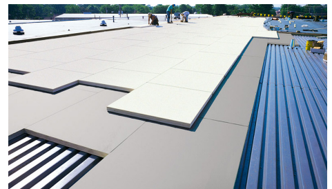
Polyiso roof insulation on a commercial building.
