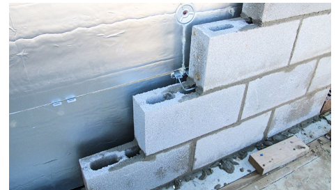
Polyiso wall insulation on a commercial building.
