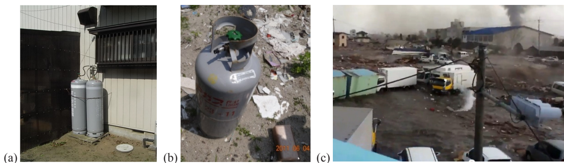
Fig. 3. Liquefied propane gas cylinders at usual situation (a) and tsunami affected situation (b), (c).
