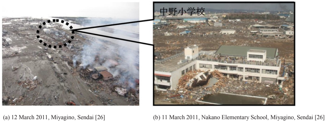
Fig. 23. Tsunami refuge building in fire risk. (a) location of elementary school and the fire; (b) elementary school with a lot of combustible materials.
