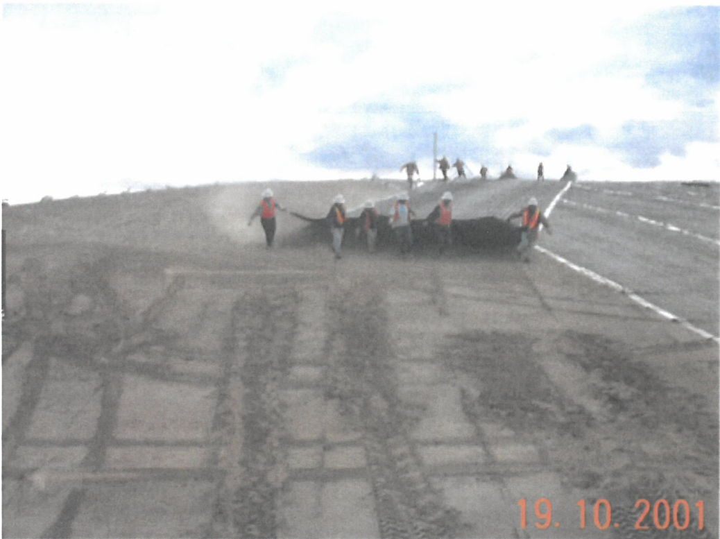
Deployment of 40 mil textured LLDPE geomembrane on west slope MSW area.
