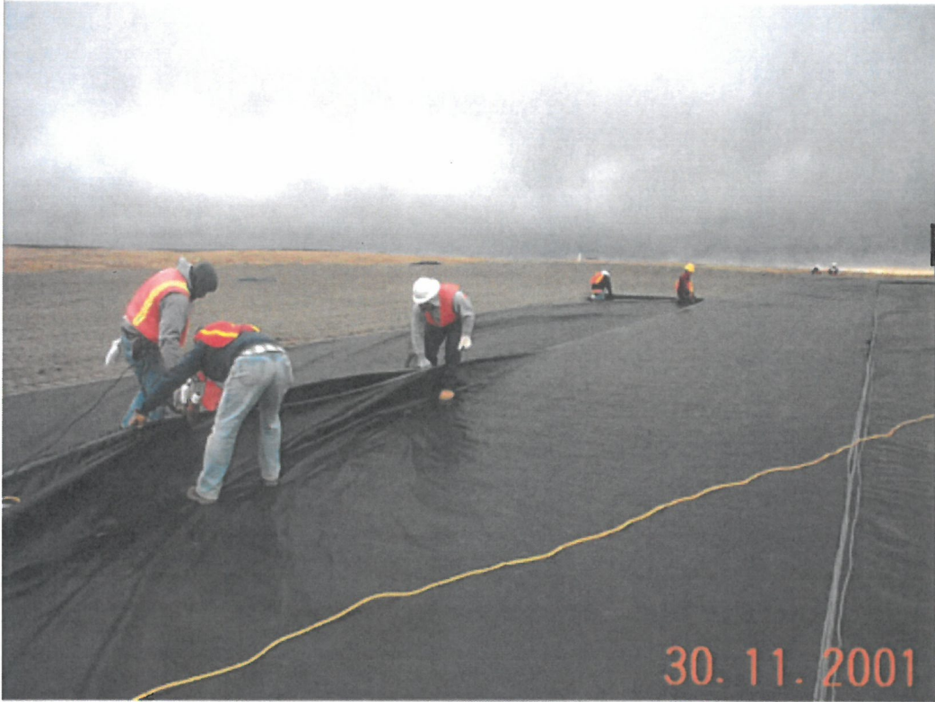
Field Lining Systems sewing geotextile.
