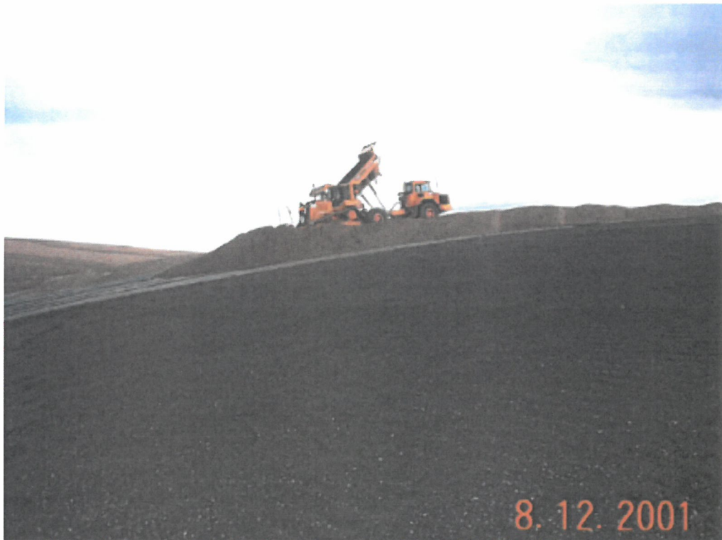
Vegetative soil layer placement on north slope of MSW area.
