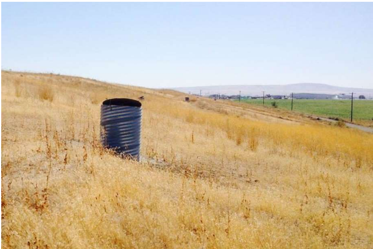
Photo of same portion of MSW Landfill cover in 2019
