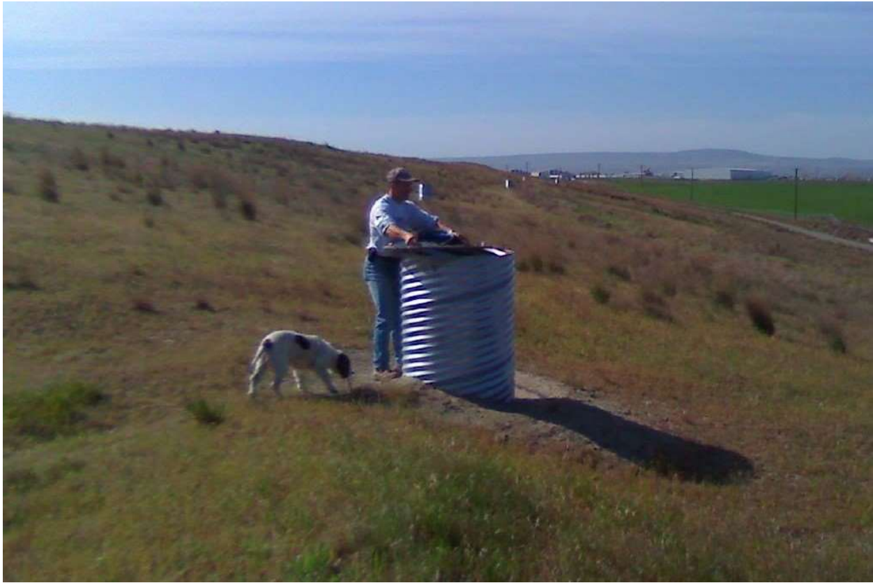
Photo of portion of MSW Landfill cover in 2010
