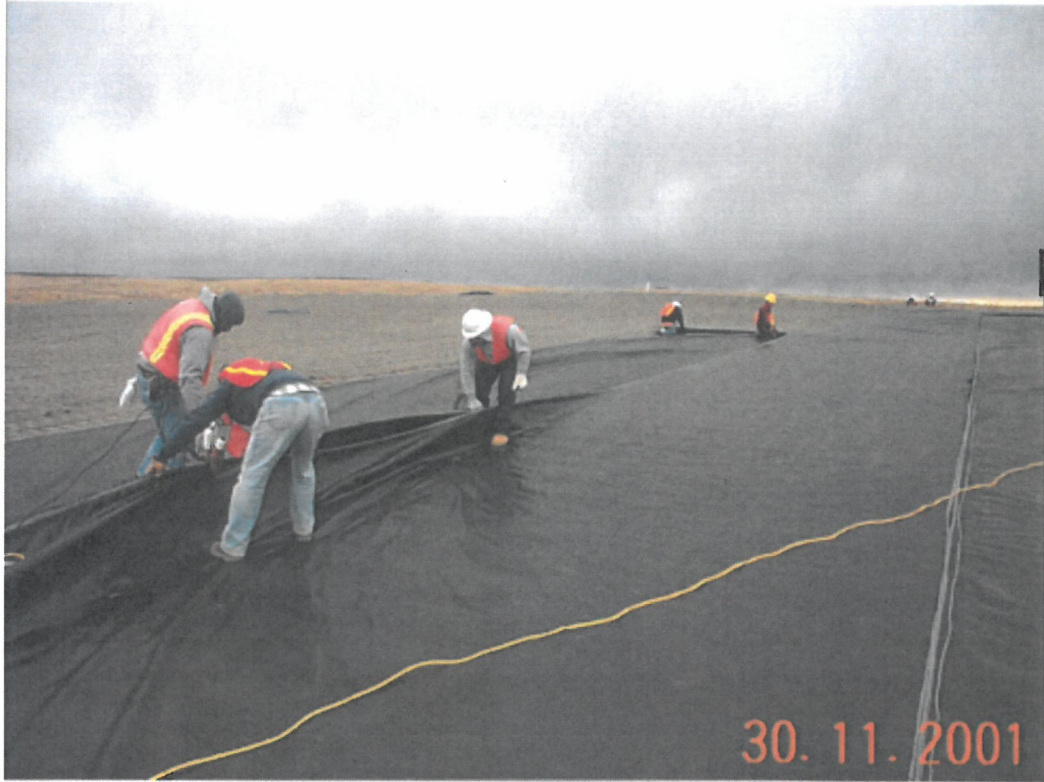
Field Lining Systems sewing geotextile.
