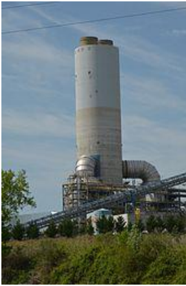
The G. G. Allen Steam Station scrubber
