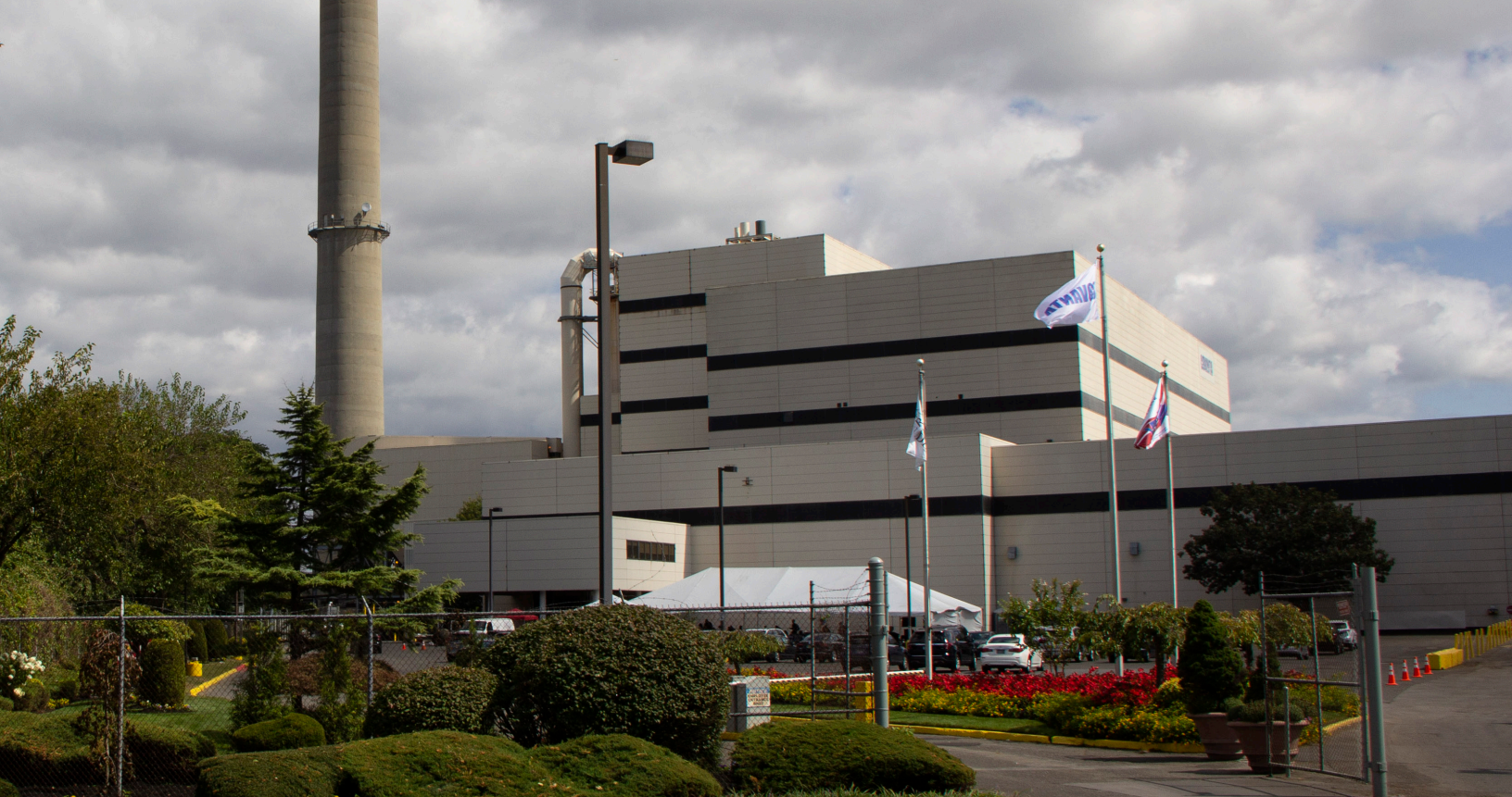
Hempstead, NY WTE Facility located 29 miles from New York City
