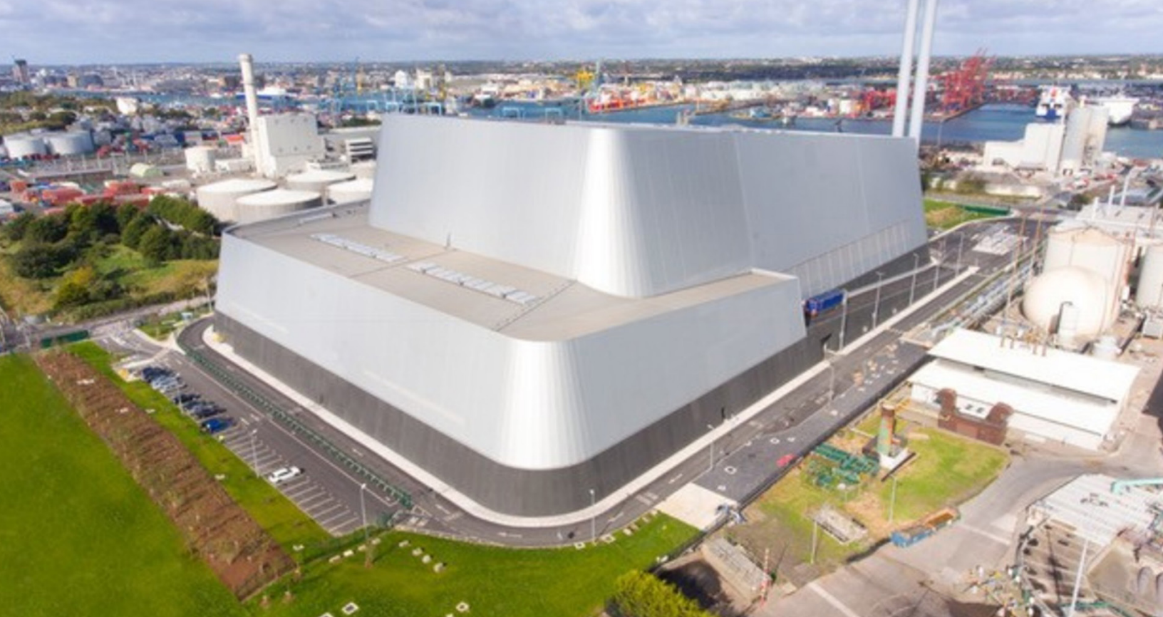
Dublin Waste-to-Energy Facility – www.dublinwastetoenergy.ie
