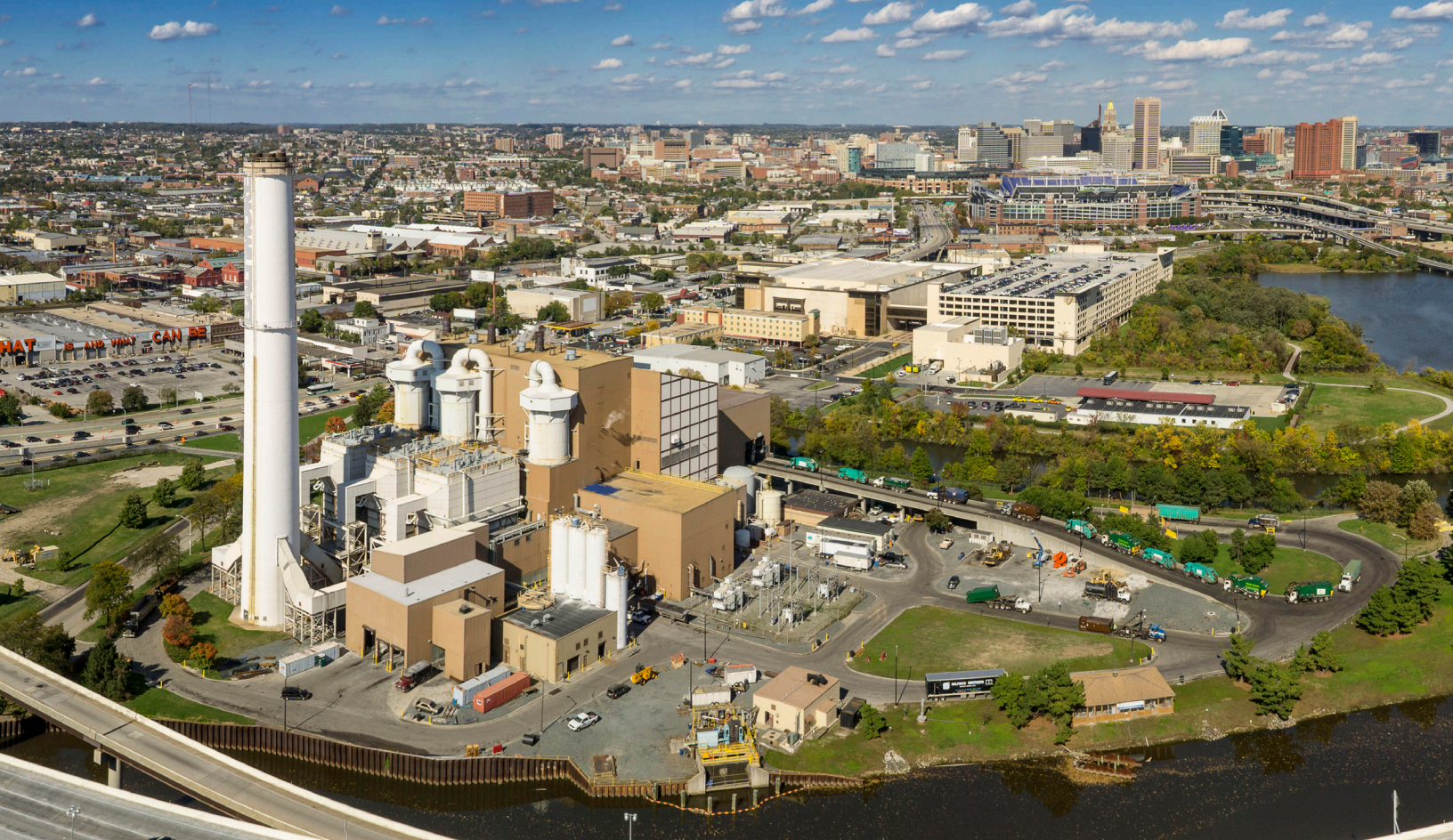
Baltimore waste-to-energy facility
