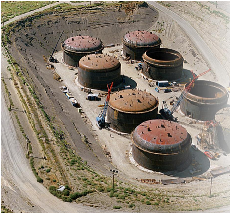
Double Shell Tanks under construction in the 1970's.
