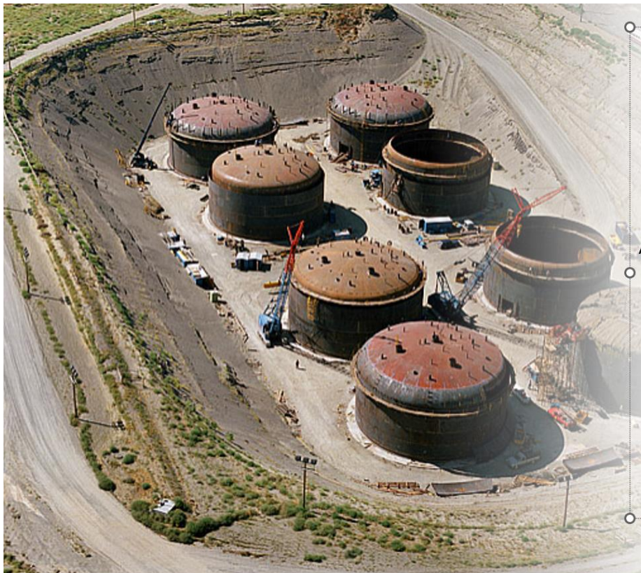
Double Shell Tanks under construction in the 1970's.
