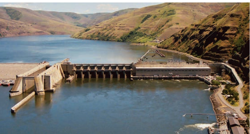
Courtesy US Army Corps of Engineers
