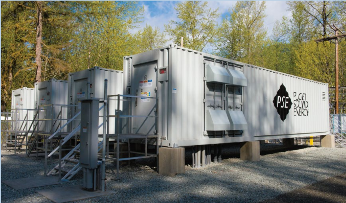
Example of a BESS interior
