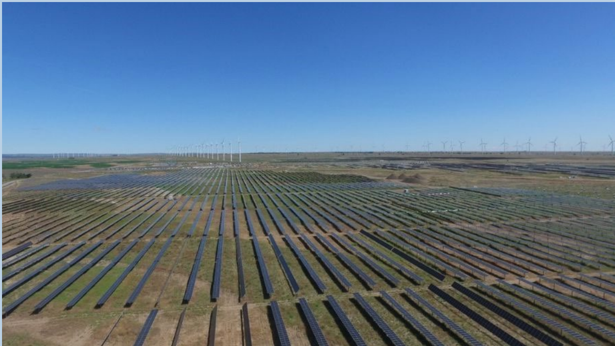
Photograph from Business Wire
