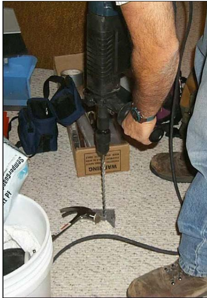
Figure D-1: Drilling through a concrete slab using a rotary hammer drill (Photo credit: EPA 2006)
