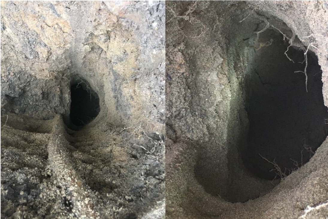
Photograph 6: View along Pipe 3 and the eastern sidewall of the tank. The tank was determined to be 4.5 feet in height. The excavation reached approximately 8 feet bgs and no groundwater or petroleum impacted soil were observed.
