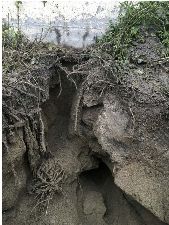
Photograph 9: View of the northern extent of the excavation area, facing north with the Jurgensen building in the background. There were no features observed extending across the property boundary.
