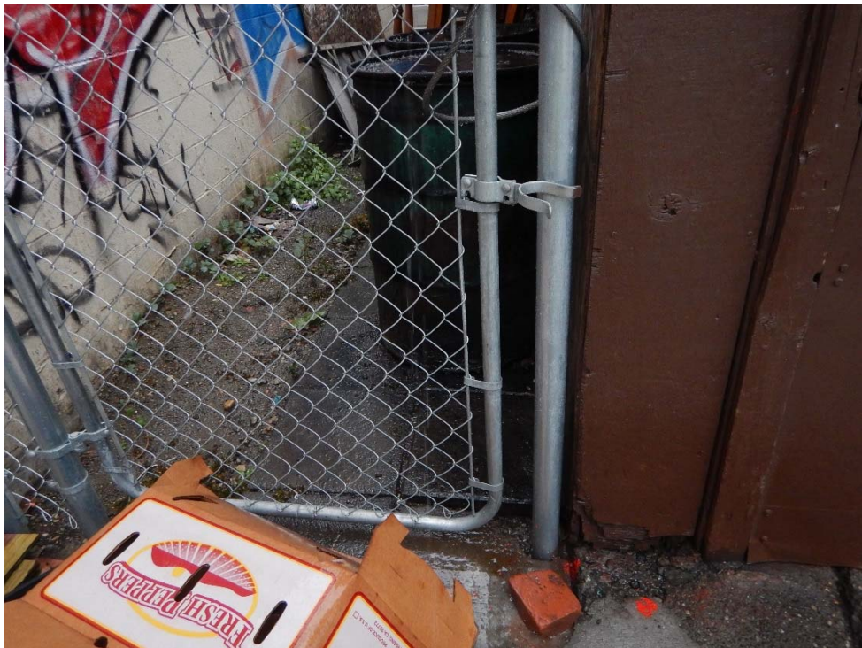
Photograph 2: View of fenced alley and Building Addition, facing east. Orange paint marks the continuation of Pipes 2 and 3 identified by the utility locator. The locate marking for Pipe 1 was located directly north of the red brick in view, but was obscured by heavy rainfall.
