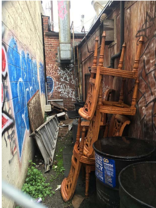
Photograph 11: View of the walkway located north-adjacent to the Building Addition, facing east. Pictured are two drums apparently used to store cooking oil.
