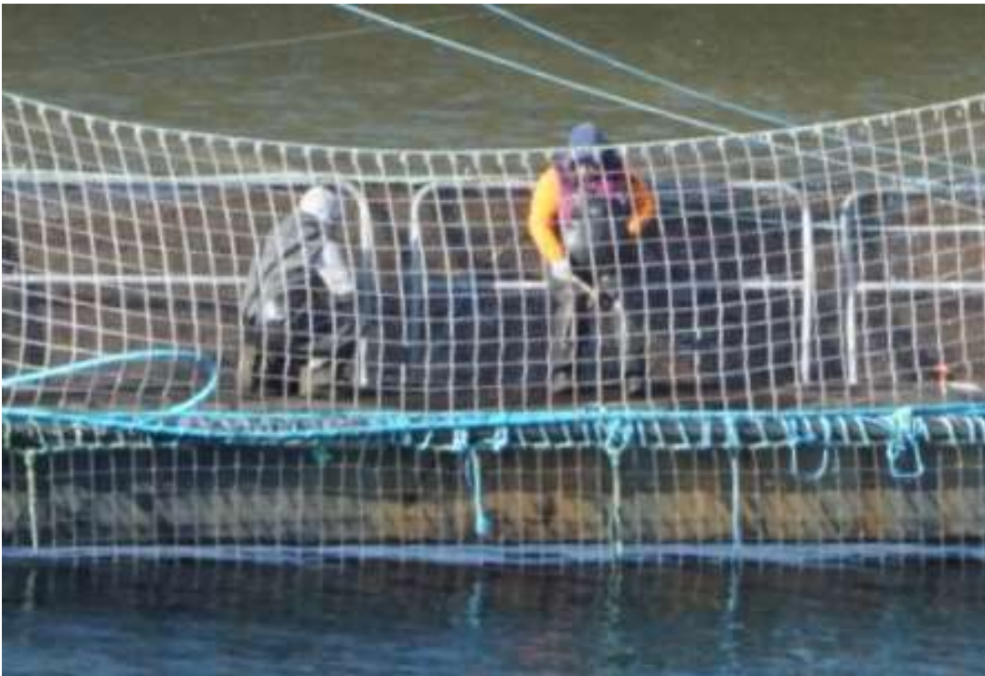
Photo of workers hammering rust off the Orchard Rocks facility 2018
