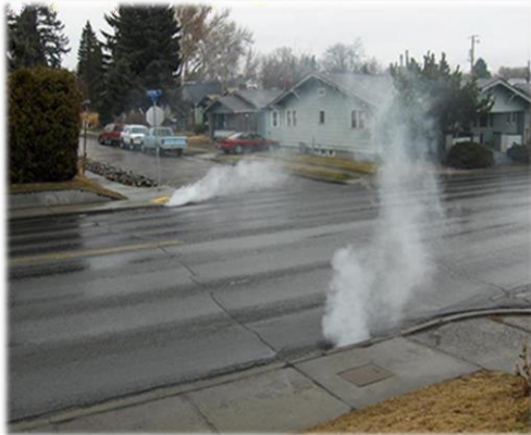
Figure 35: Illicit connection smoke testing.
