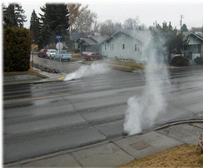
Figure 35: Illicit connection smoke testing.
