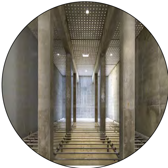
Interior of BIOSTYR Cell
