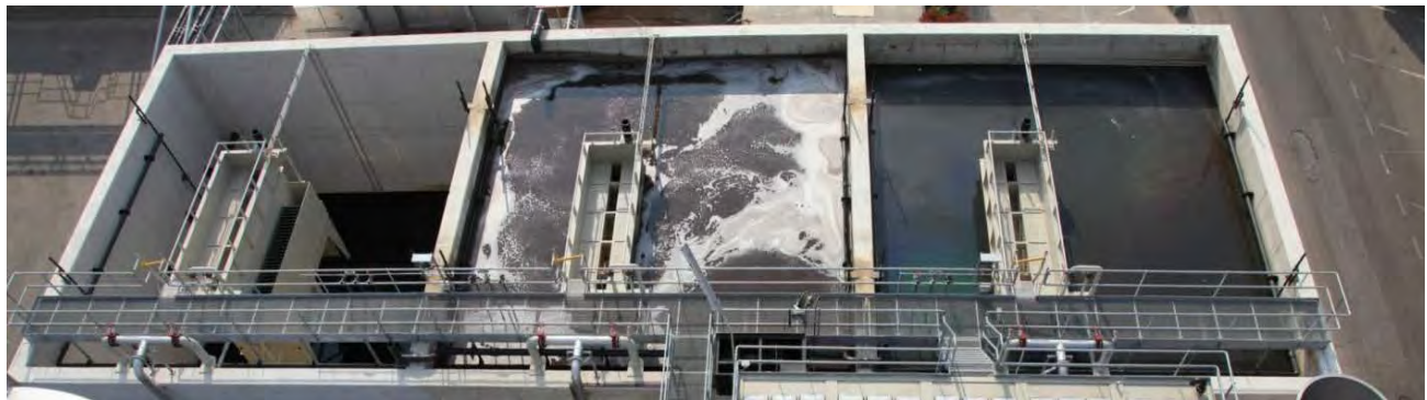
Figure:1 Modular AnammoPAQ® setup at Rendac, The Netherland (13,000 lds N/day)
