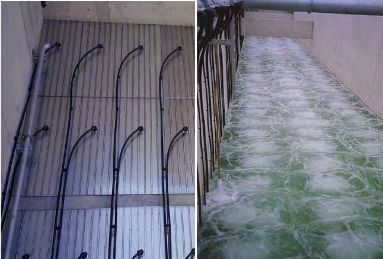
FIGURE 8 – MESSNER PANEL INSTALLED / AERATION PATTERN TEST
