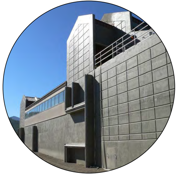
10 MGD Tahoe-Truckee SD BIOSTYR - Truckee, CA
