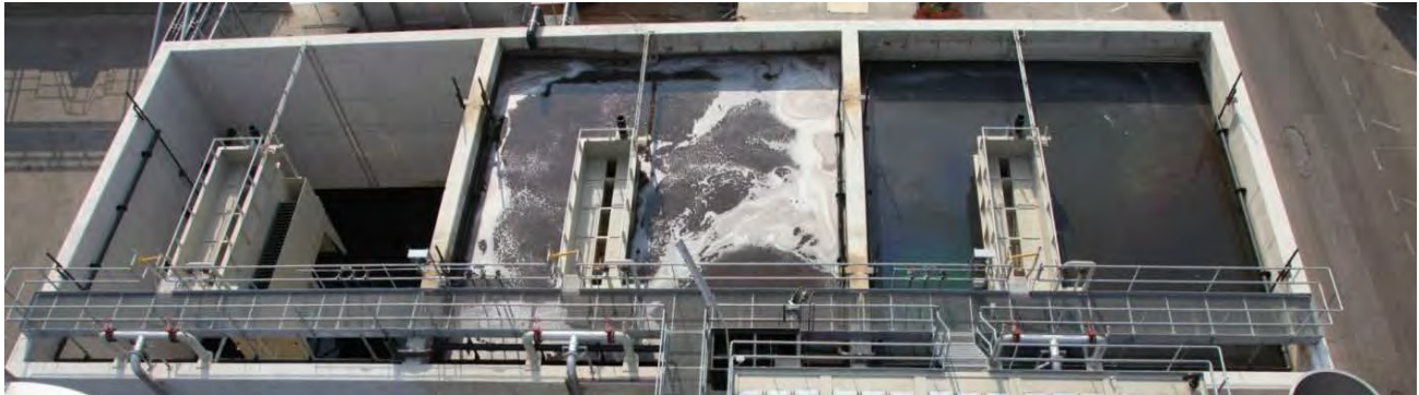
Figure:1 Modular AnammoPAQ ® setup at Rendac, The Netherland (13,000 lds N/day)
