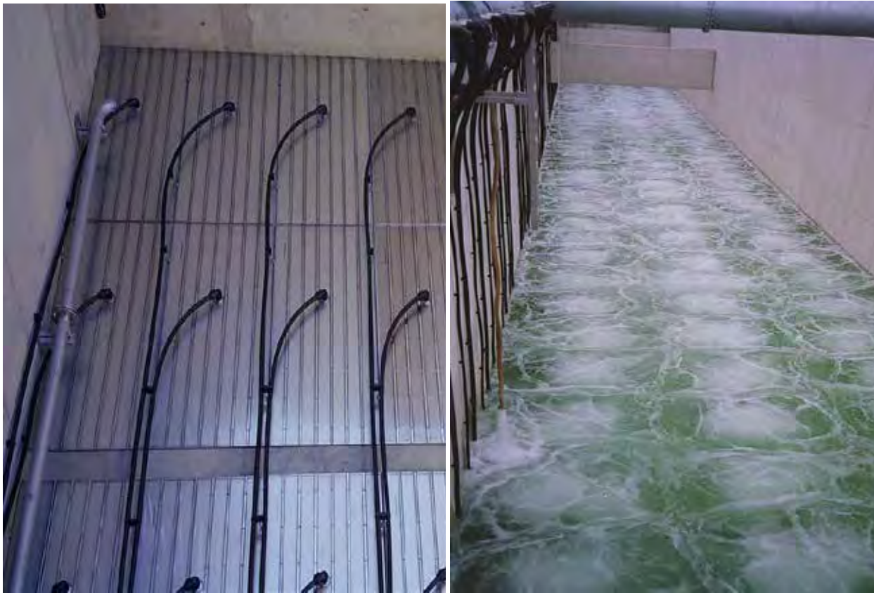
FIGURE 8 – MESSNER PANEL INSTALLED / AERATION PATTERN TEST
