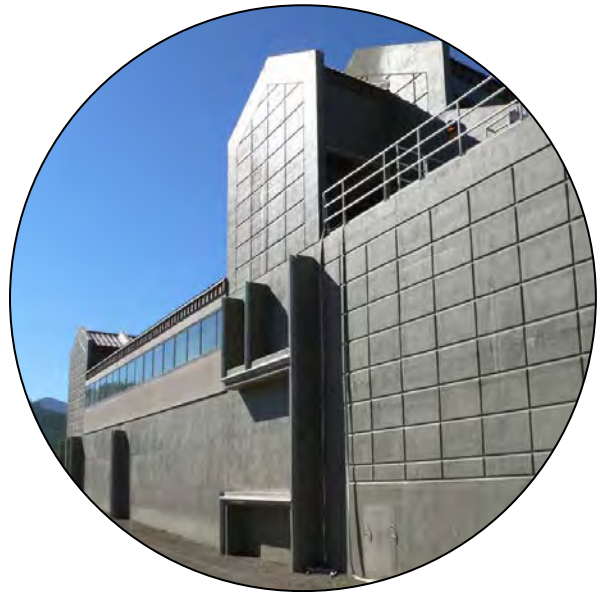
10 MGD Tahoe-Truckee SD BIOSTYR - Truckee, CA
