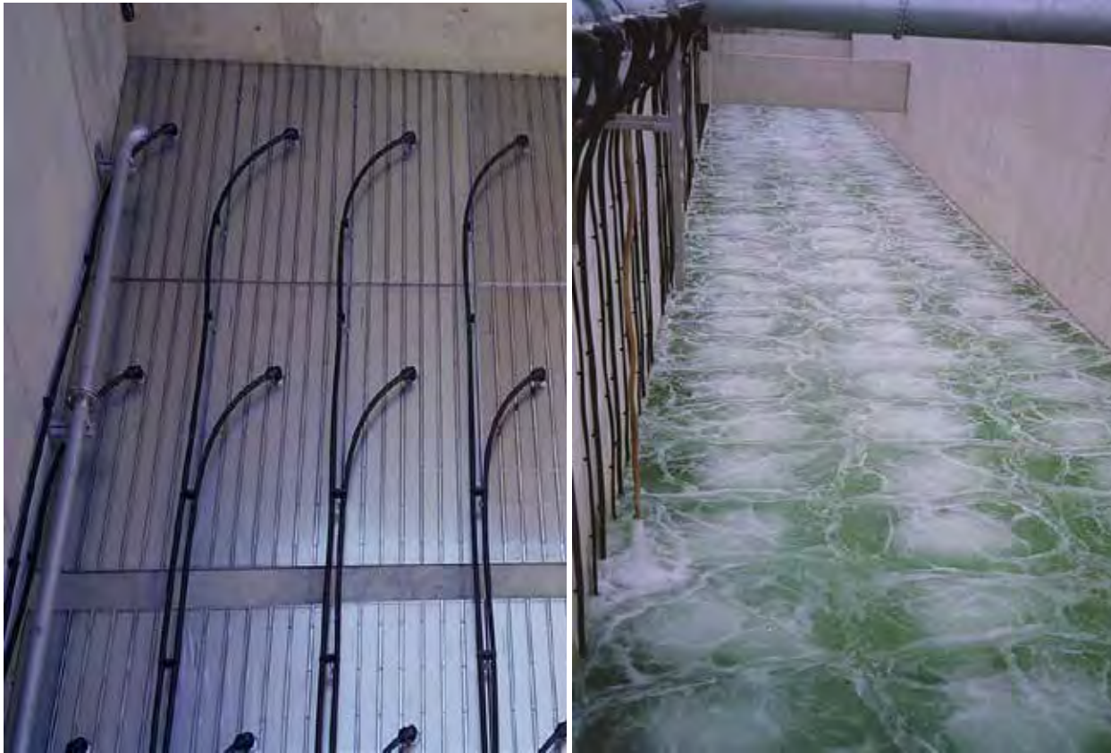
FIGURE 8 – MESSNER PANEL INSTALLED / AERATION PATTERN TEST
