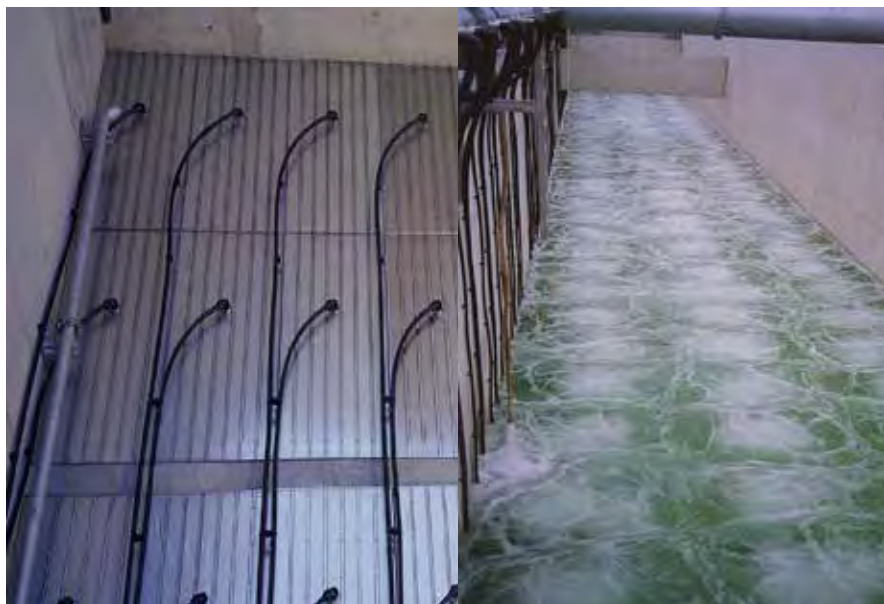
FIGURE 7 – MESSNER PANEL INSTALLED / AERATION PATTERN TEST
