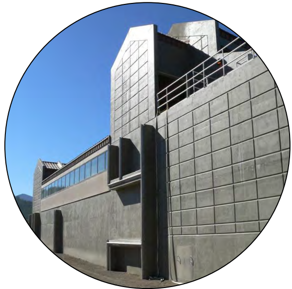
10 MGD Tahoe-Truckee SD BIOSTYR - Truckee, CA
