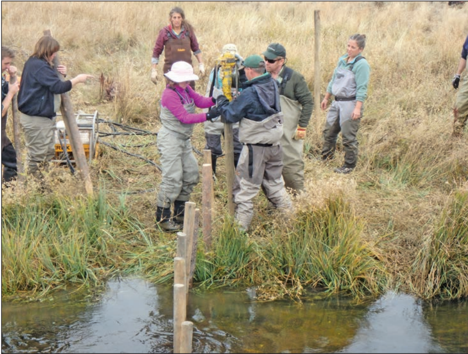
Figure 3—Groups learn about installing beaver dam analogues on workshops and field trips, such as this one on Bridge Creek in Oregon.
