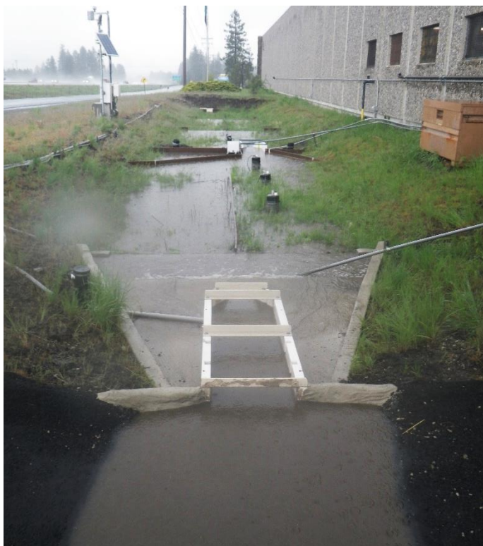
Figure 4. Example of a compost-amended biofiltration swale. Stormwater is filtered as it flows along the grass in the swale and infiltrates into the topsoil and compost. Photo: Washington State Department of Transportation.
