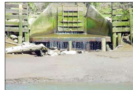
Combined sewer overflow (CSO) outfall (photo courtesy of WADOE)
