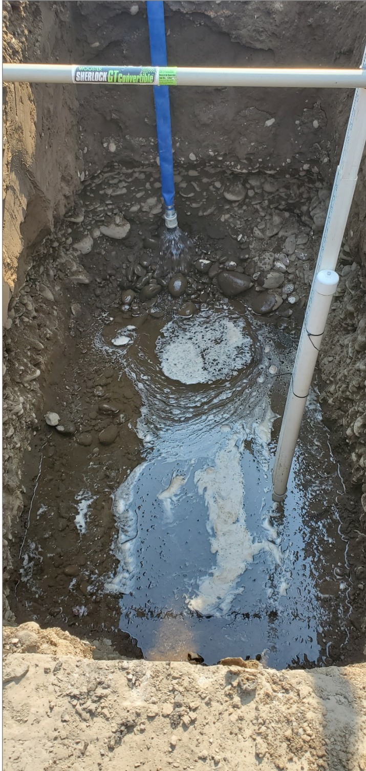
Photograph 8. INF #4 small-scale PIT. (July 21, 2021)
