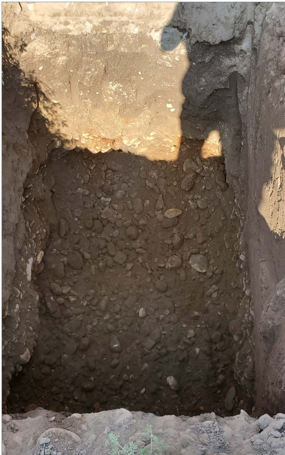
Photograph 5. INF #3 small-scale PIT. (July 23, 2021)
