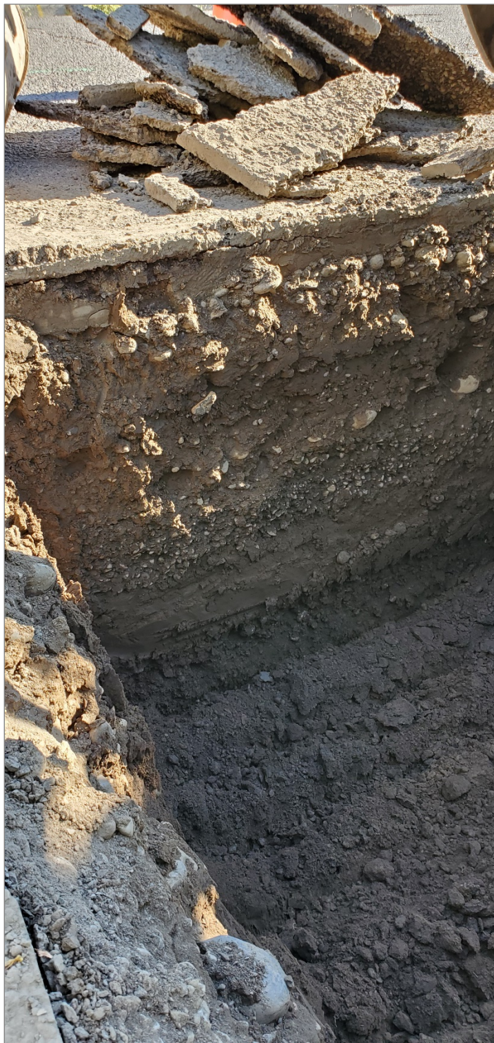
Photograph 1. INF #1 small-scale PIT. (July 22, 2021)
