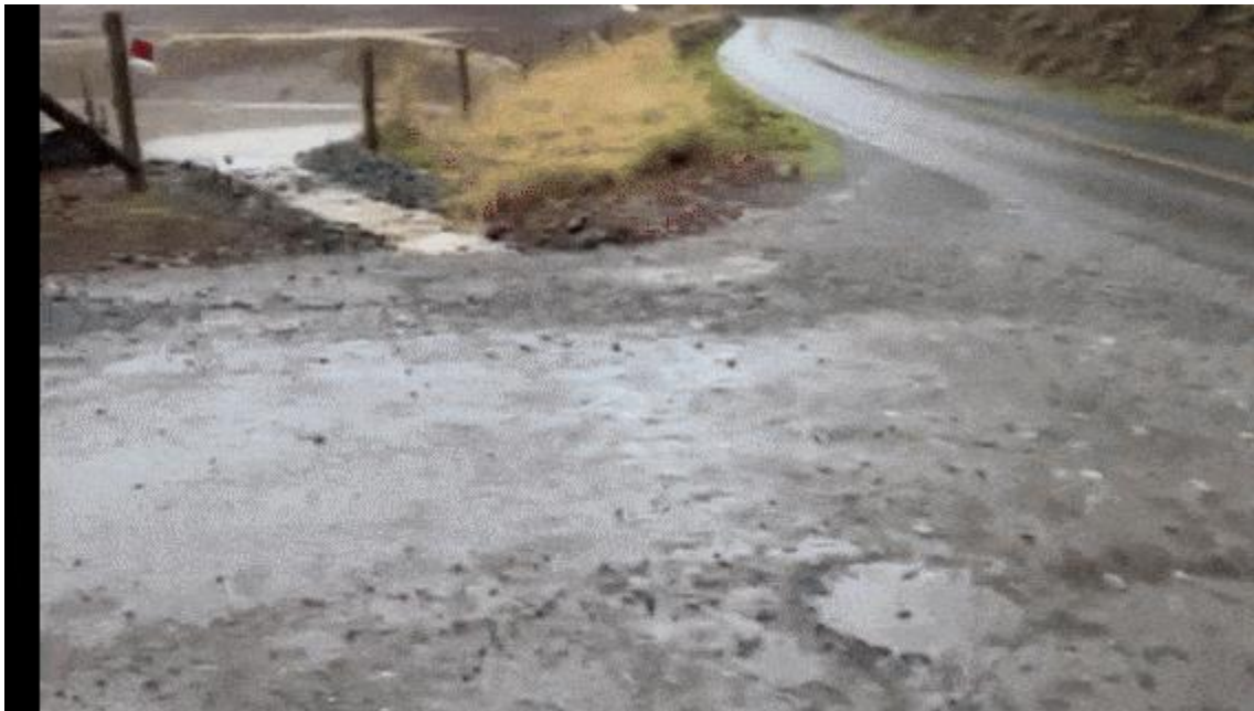
Figure 2: Video by neighbor Joshua Lindquist on or about December 5, 2023 showing improperly constructed Edelbrock sediment pond blowout and turbid water release. The sediment pond was not constructed in accordance with SWPPP drawings approved by Snohomish County PDS who in turn refused to take any enforcement action. There was no CSGP issued by Ecology prior to commencement of land disturbing activities.
