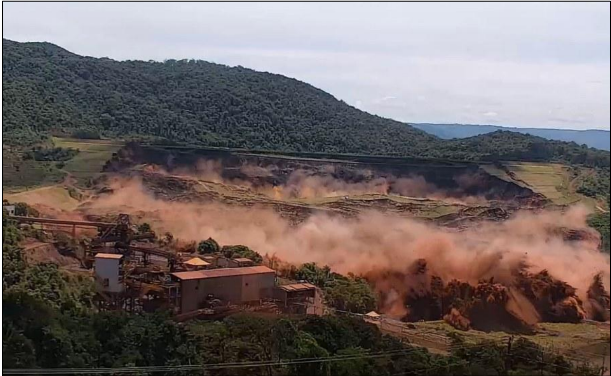
Figure 5. The failure of the upstream tailings dam at the Córrego do Feijão mine near Brumadinho, Brazil, on January 25, 2019, which resulted in 272 deaths, including the deaths of 258 mineworkers, was a watershed moment in the global awareness of the danger of the upstream construction method. However, in the five decades preceding the Brumadinho disaster, there were already numerous cautions and prohibitions regarding the use of the upstream method in guidance documents and regulations. Photo from Robertson et al. (2019).
