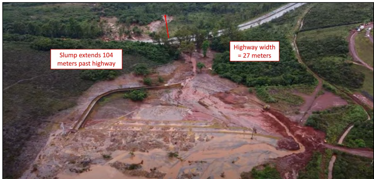
Figure 15a. Based on the highway width of 27 meters, the slump at the filtered tailings storage facility at the Pau Branco mine in Brazil on January 8, 2022 (see Fig. 14), extended for 104 meters past Highway BR-40. Highway width was measured from Google Earth image from June 29, 2022 (see Fig. 15b). Still image at 0:38 of drone video (Observatório da Mineração [Mining Observatory], 2022).
