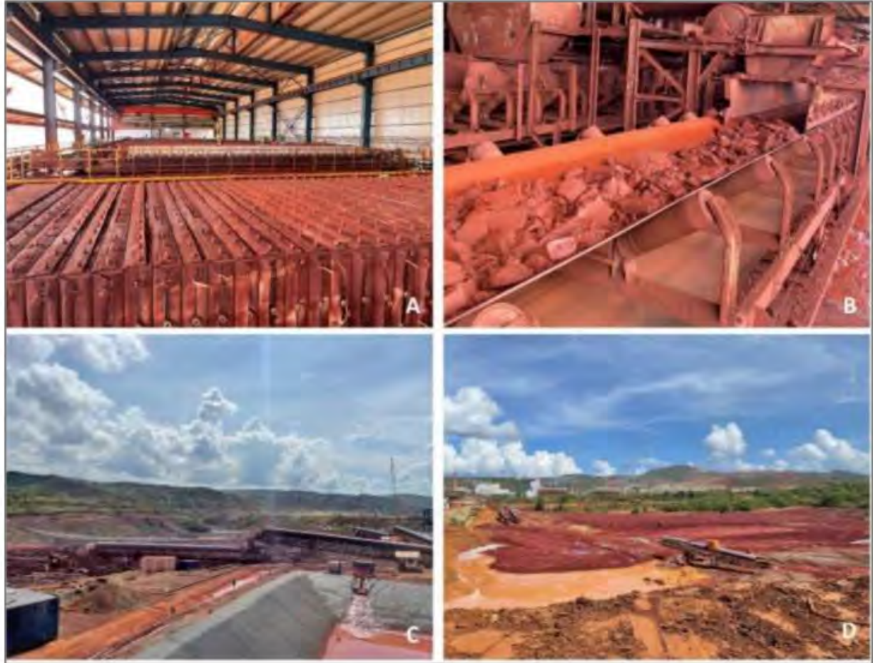
Figure 7-6: Dry stack tailings facility operation
