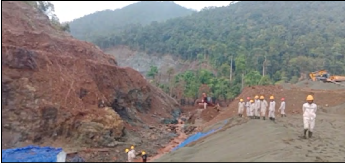
Figure 42a. The collapse of the filtered tailings storage facility of PT Qing Mei Bang (QMB) New Energy Materials in the Indonesia Morowali Industrial Park (see Figs. 3, 23, 24, and 41a) on March 21, 2025, resulted in the burial of four workers with three fatalities and one survivor. The four workers were employees of PT Morowali Investasi Konstruksi Indonesia (MIKI), which is a contractor of PT QMB New Energy Materials. Because of the similarity with Fig. 40a, it is not clear as to whether the filtered tailings storage facilities of PT HYNC and PT QMB are actually separate facilities. Still image at 0:12 from video shared by mineworker.
