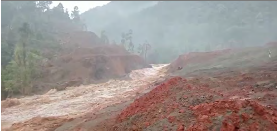
Figure 40a. Liquefied tailings flow through a breach of the filtered tailings storage facility of PT Huayue Nickel Cobalt (HYNC) in the Indonesia Morowali Industrial Park (see Figs. 3, 24, and 41a-b) on March 16, 2025. Still image at 0:00 of 9-second video by mineworker at PT HYNC. Photo also available in Business & Human Rights Resource Centre (2025a) and Moore (2025).
