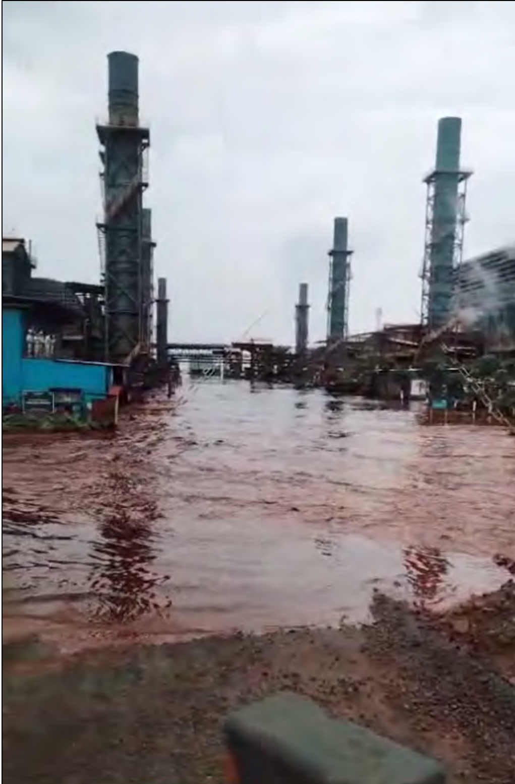
Figure 40c. Liquefied tailings from the failure of the filtered tailings storage facility of PT HYNC plus flood water from the Bahodopi River (see Figs. 40a-b) overflow onto the site of PT Fajar Metal Industry (FMI) on March 16, 2025 (see Figs. 23-24). Still image at 0:03 of 10-second video by mineworker.
