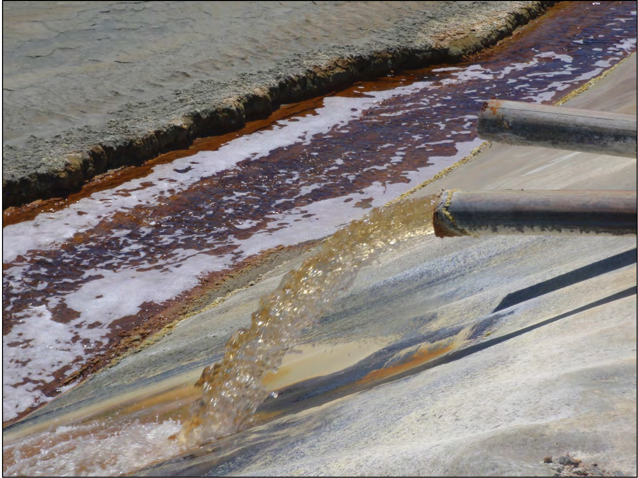
Figure 8b. A mixture of water and tailings with a solids content of 35% by mass is hydraulically discharged into the tailings pond from the crest of the Cobre dam at the Atalaya Mining Riotinto mine in Andalusia, Spain (see Fig. 7). Because of the lack of compaction, the loosely-packed tailings are susceptible to liquefaction (see Fig. 10). Photo taken by the author on June 21, 2019.
