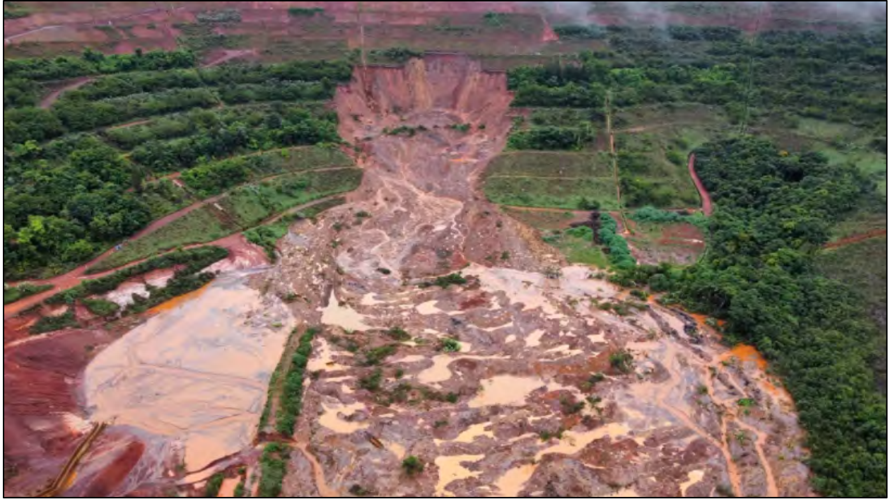
Figure 14. A 48-meter-high filtered tailings stack collapsed at the Pau Branco iron-ore mine in Brazil on January 8, 2022. Although filtered tailings are regarded as the Best Available Technology at the present time (Independent Expert Engineering Investigation and Review Panel, 2015; Morrill et al., 2022), the use of filtered tailings technology is not a license to ignore every other aspect of safety. Photo from Angelo (2022).
