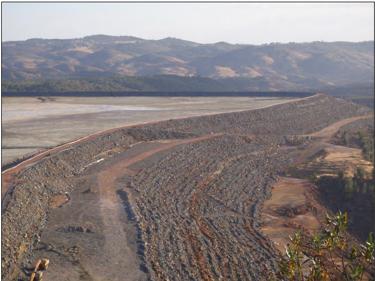
Figure 7. In conventional tailings management, wet tailings are permanently stored behind a dam constructed from waste rock, the coarser fraction of the tailings, or rockfill or earthfill that is available on the mine site. Photo of the Aguzadera dam at the Atalaya Mining Riotinto mine in Andalusia, Spain, taken by the author on June 19, 2019.
