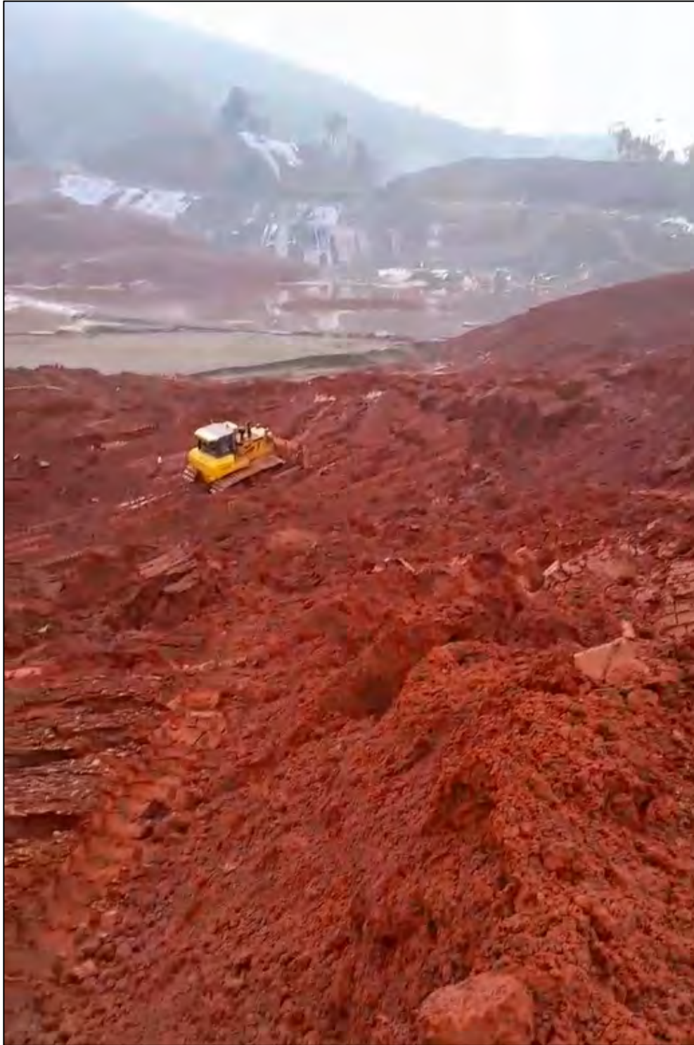
Figure 44. On April 30, 2025, a landslide occurred at the filtered tailings storage facility of PT Qing Mei Bang (QMB) New Energy Materials project in the Indonesia Morowali Industrial Park (see Figs. 3, 23, and 24), Still image at 0:12 of 30-second video by mineworker.
