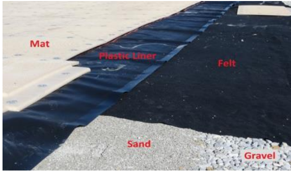
Well Pad Liner and Subbase Materials
