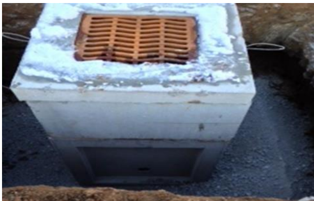
Catch Basin Installed before Backfill
