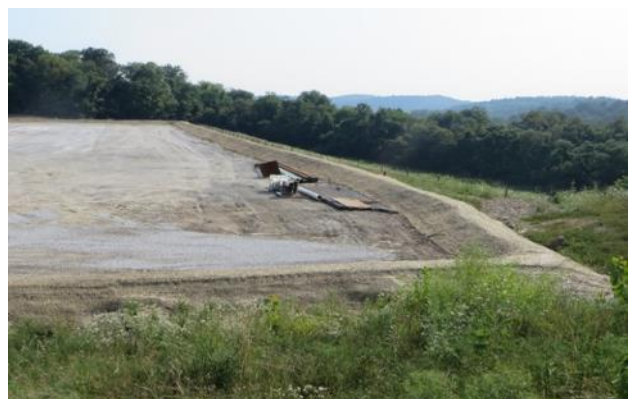
Perimeter Catch Basin
