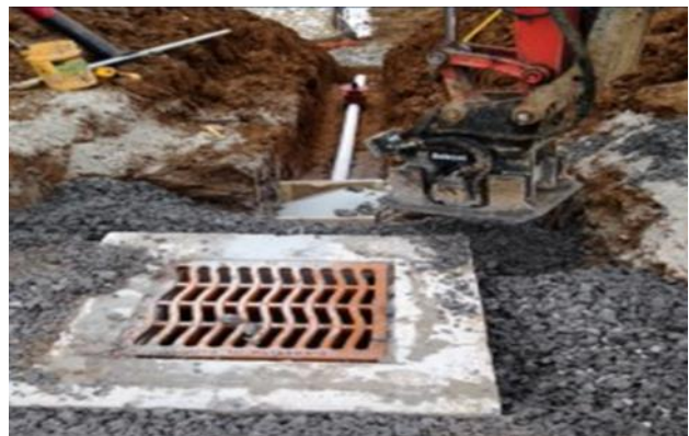
Compacting Backfill around Catch Basin
