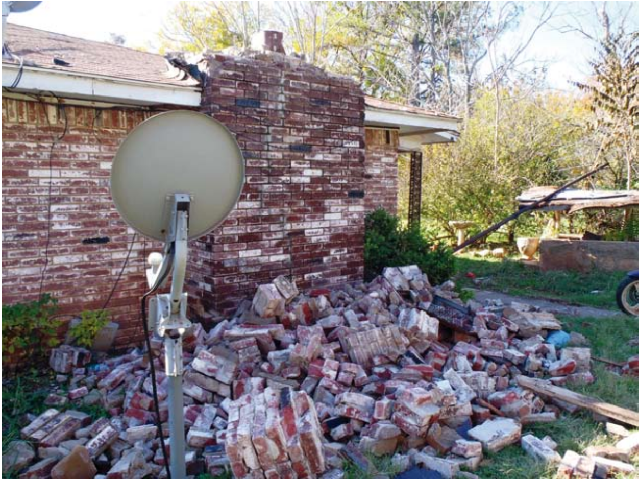
Earthquake damage in Oklahoma in 2011 linked to underground wastewater injection. Photo: Brian Sherrod/United States Geological Survey
