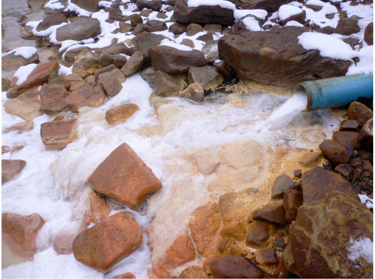
Figure 3. Effluent Outfall on Blacklick Creek [Picture taken by Kyle Ferrar, December 10, 2010, at location (40.481°N, 79.169°W)]
