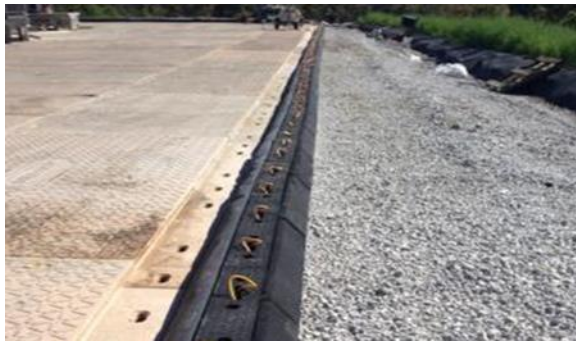
Well Pad Liner Berm
