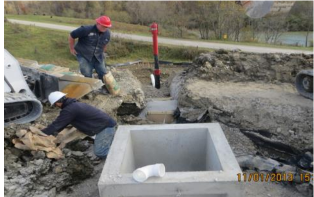
Bentonite Being Placed around Anti-Seep Collars
