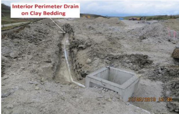
Perimeter Drain with Perforated Pipe Trench
