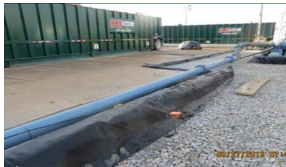
Grounding Rod Outside Containment
