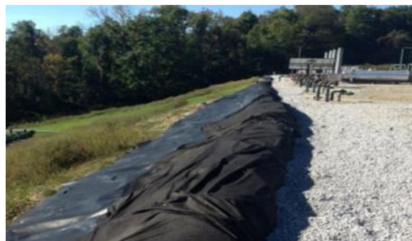
Perimeter Berm Liner and Geofabric
