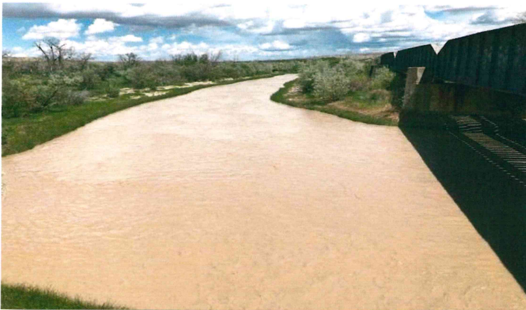
Photo 3. View of Badwater Creek from Bonneville train bridge. June 18, 2019.
