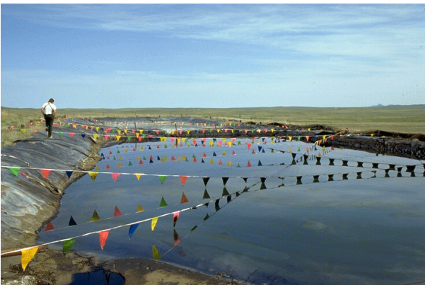
Figure A-3. Flagging is not effective at deterring birds and preventing wildlife mortality in oil pits.
