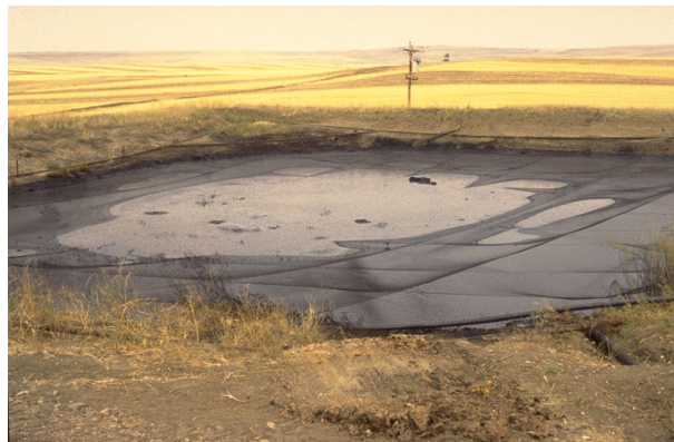
Figure A-5. Heavy snow loads can cause netting to sag into the oily fluid. Birds can land in the exposed fluid and become entrapped. Routine maintenance is necessary to keep the net from sagging into the pit.
