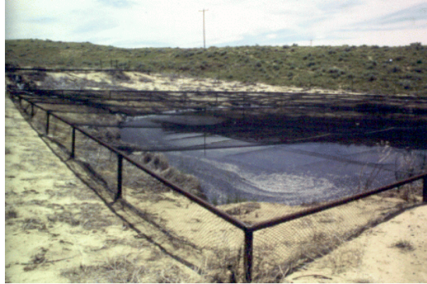
Figure A-4. Properly installed netting will exclude most wildlife from oil pits. Netting requires intensive maintenance to retain its effectiveness.
