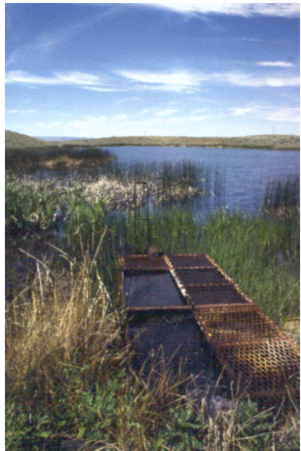
Figure A-10. Pond created by oil field produced water discharge in Natrona County, Wyoming. Discharge point (metal box) is shown in the foreground.
