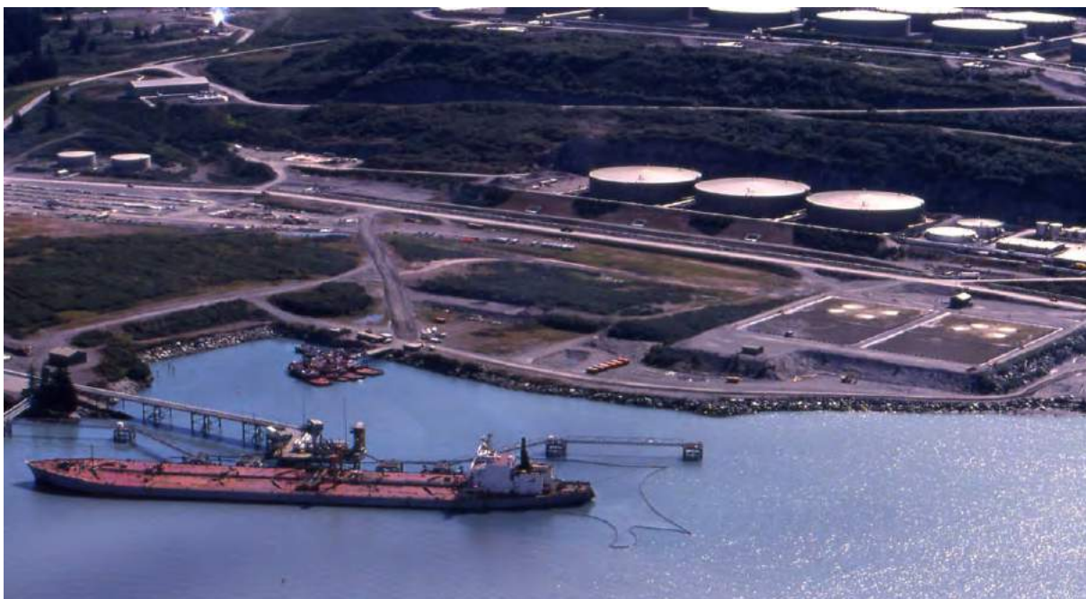
Valdez Marine Terminal in 1989. (State Archives)
