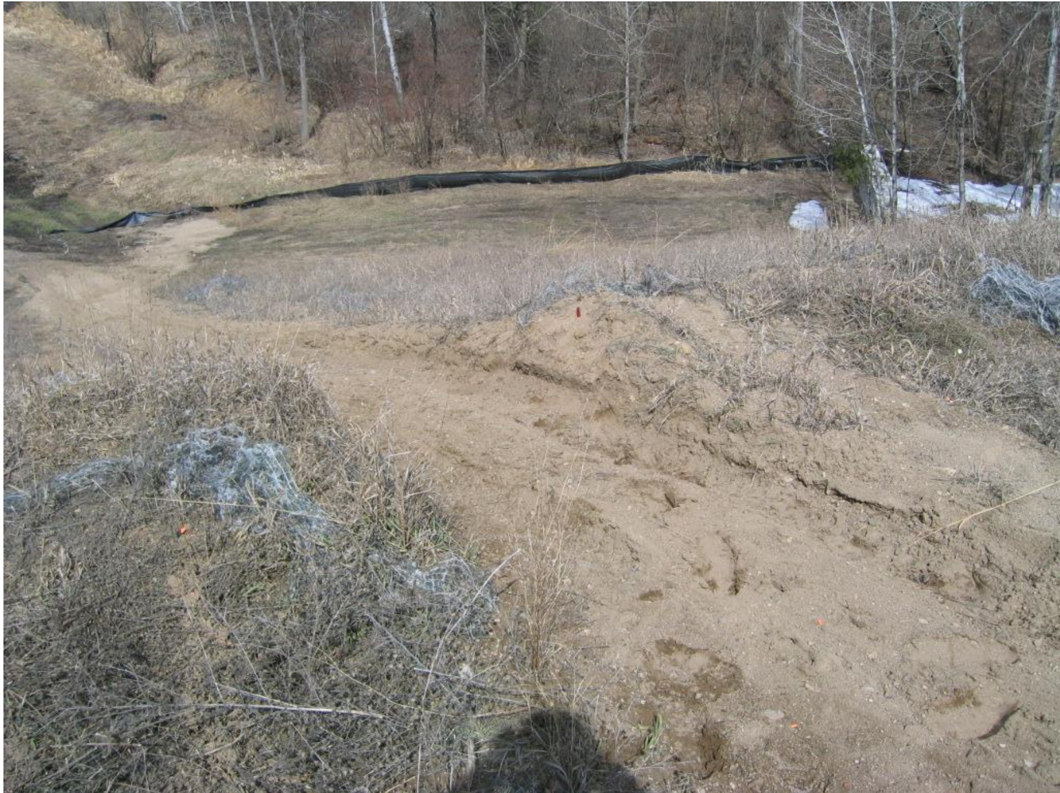
ATV traffic up and down Clearwater River bluffs through slope-breakers constructed to prevent erosion on Terrace III project.
