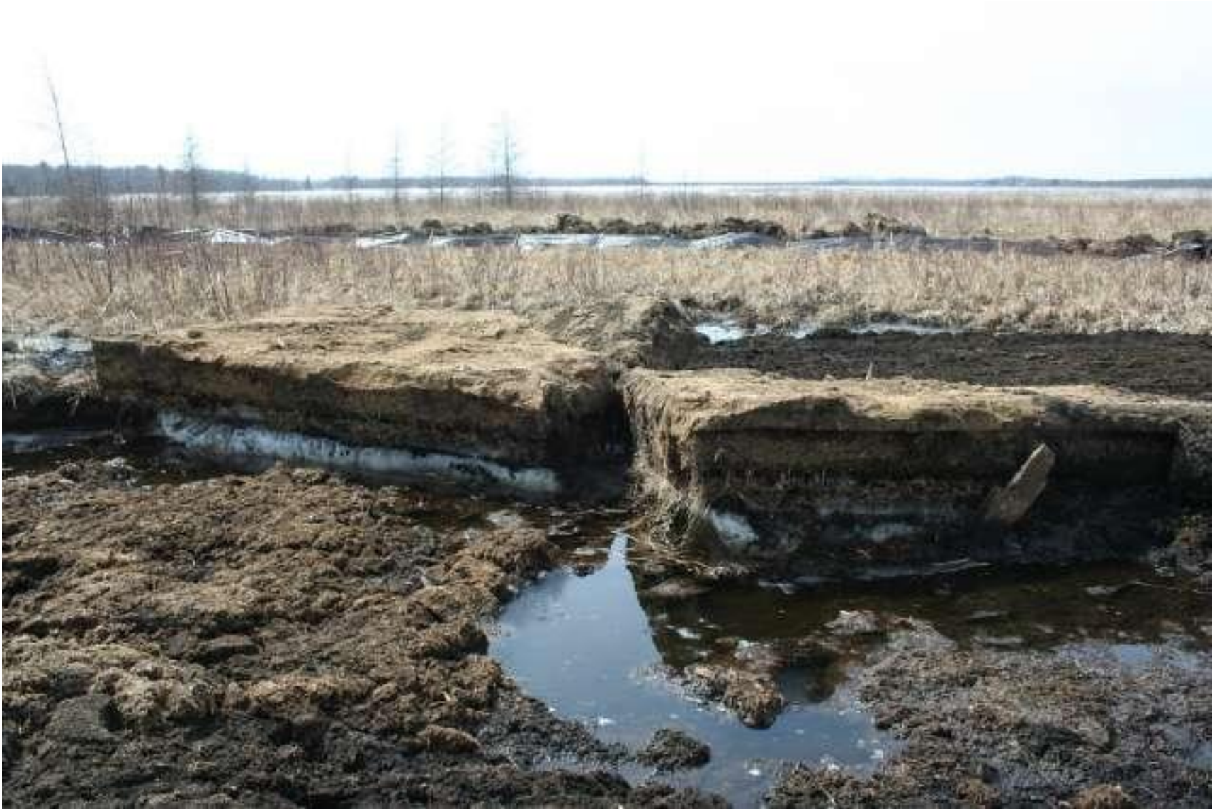
Blocks of driven-in ice on W side of ROW off trench, Mud Lake.
