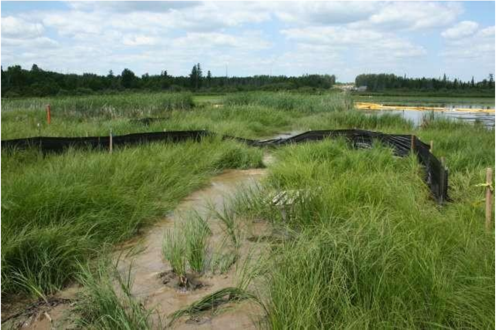
Drilling mud over HDD within S side of Hay Creek.
