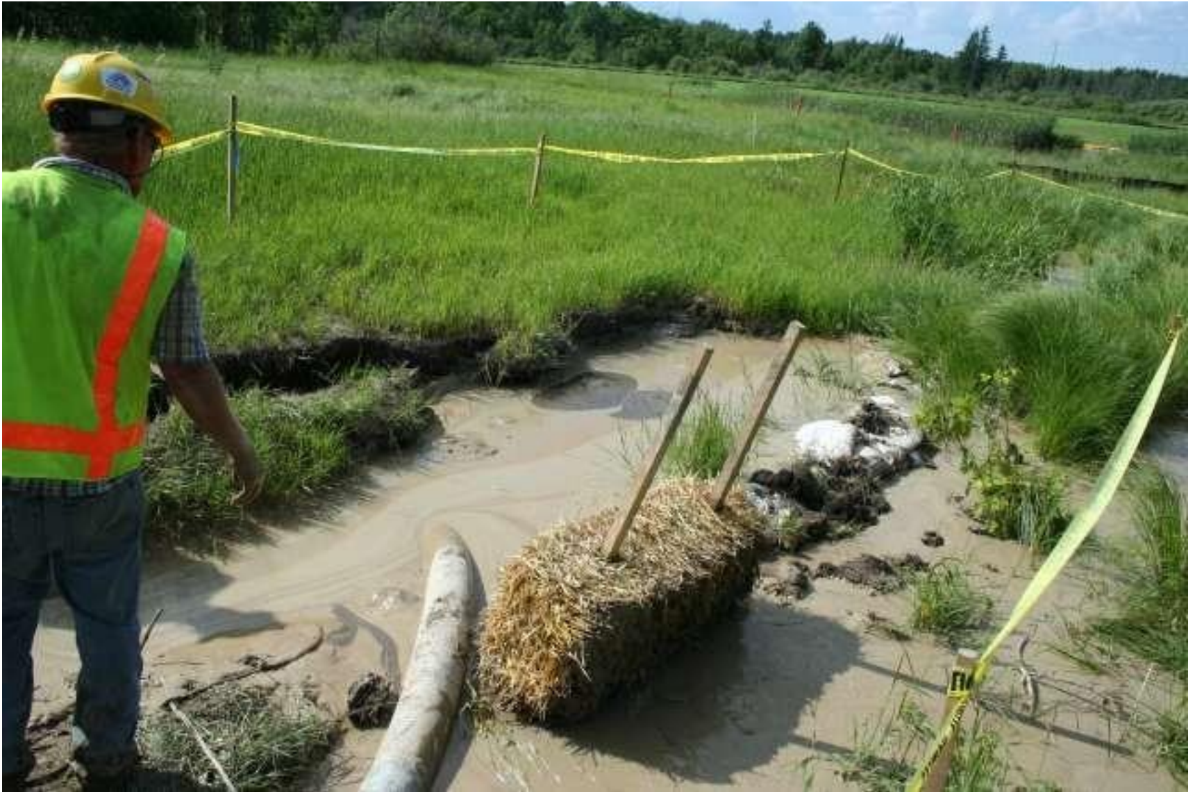
Frac bubbling up within containment over depression of HDD.
