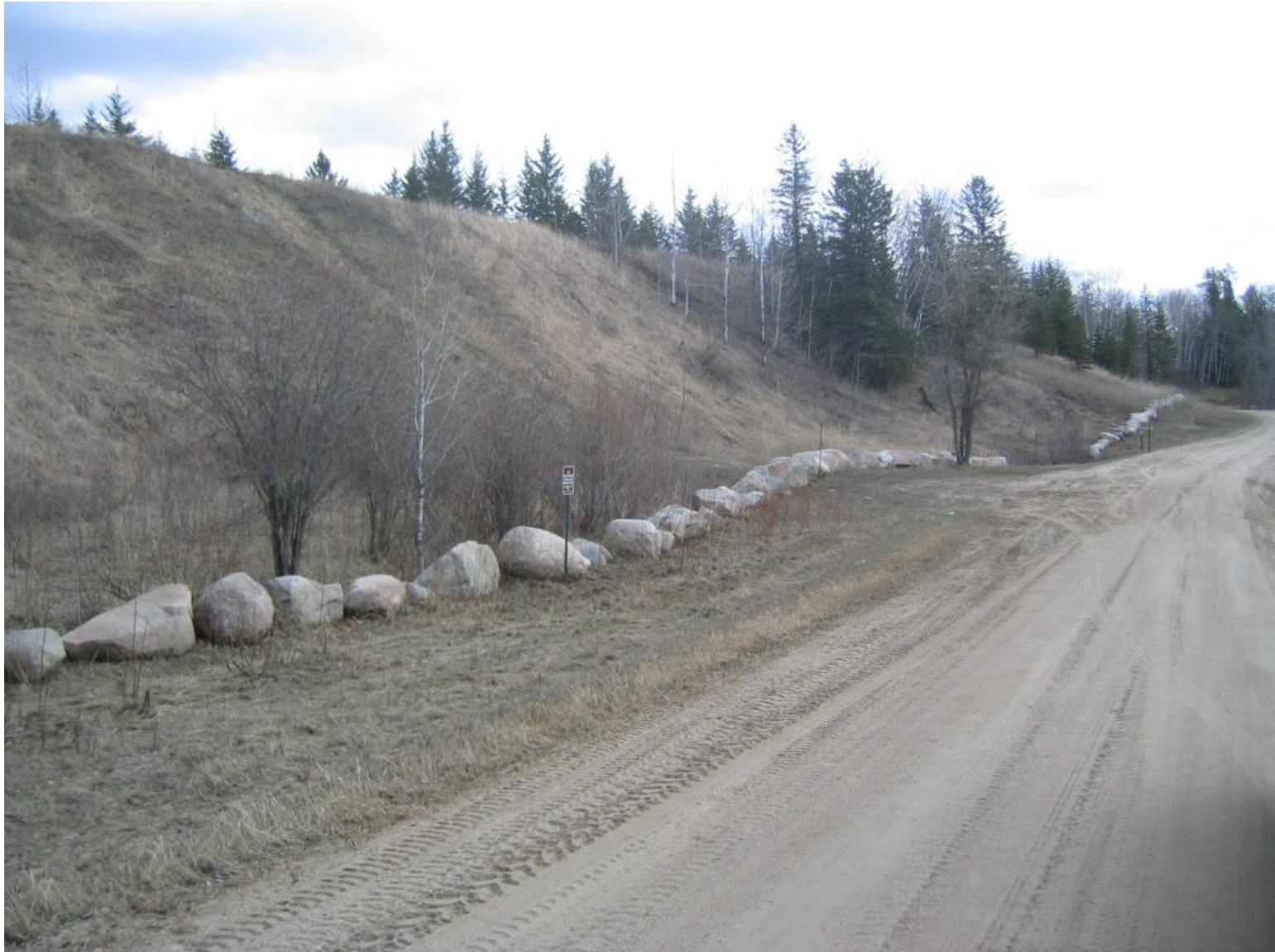
Site is adjacent to Clearwater River by railroad grade, which is now a motorized OHV recreational trail. Boulders placed at base of slope to impede ATV off-trail use
