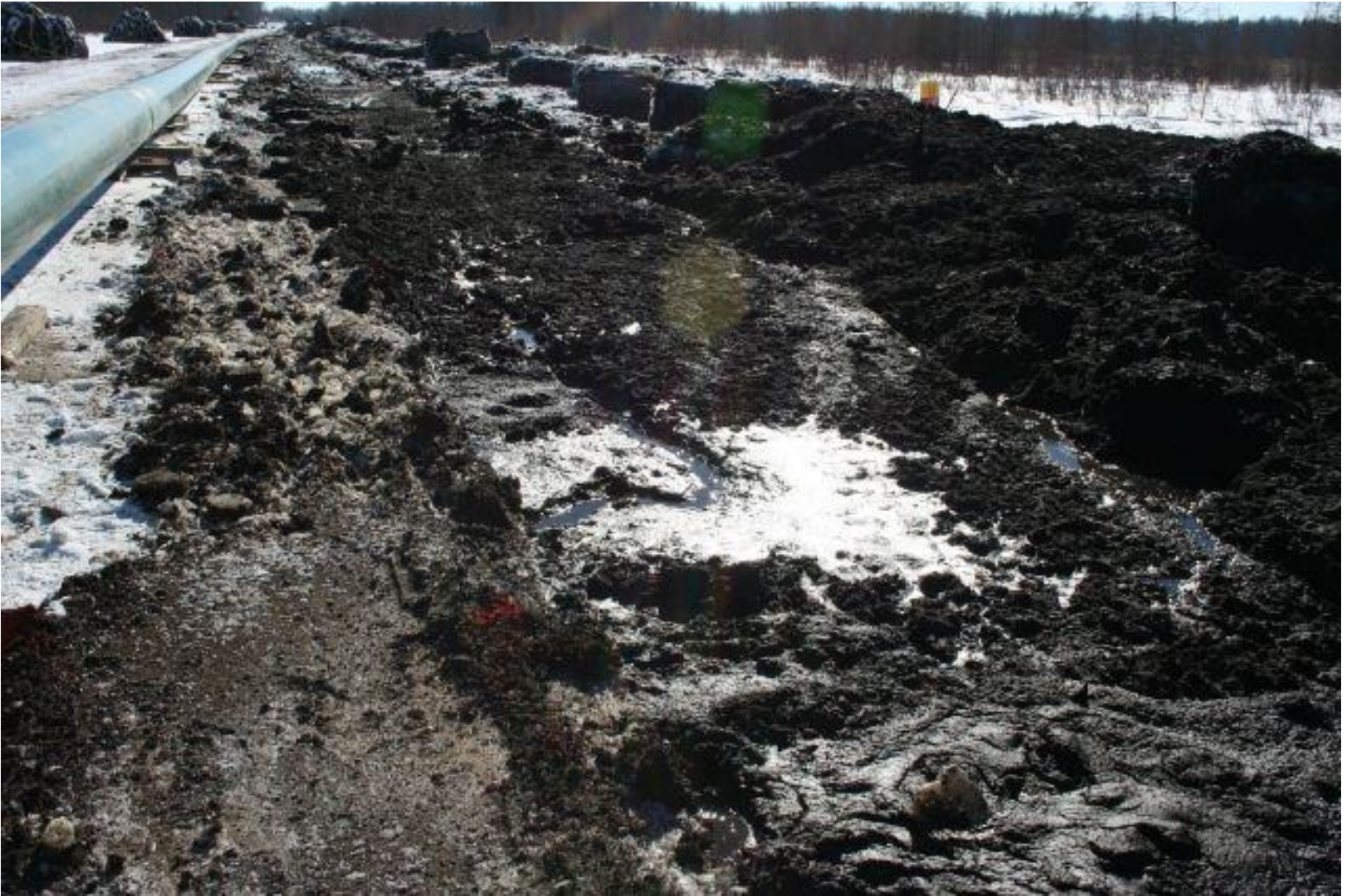
Water, ice slush and peat soil slurry refills trench, Mud Lake.
