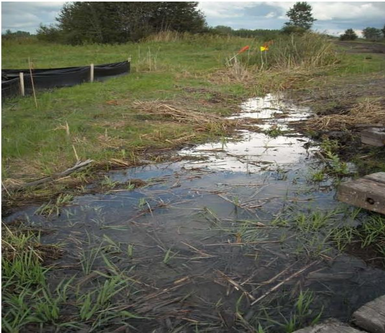
MP 845.70, Wetland W-845E, Frac-out cleanup, view east.
