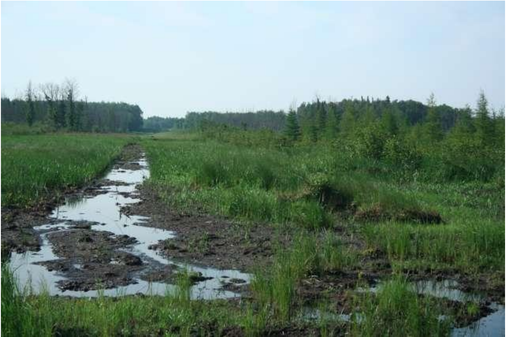
From N, trench and piles of spoil to Mud Lake.
