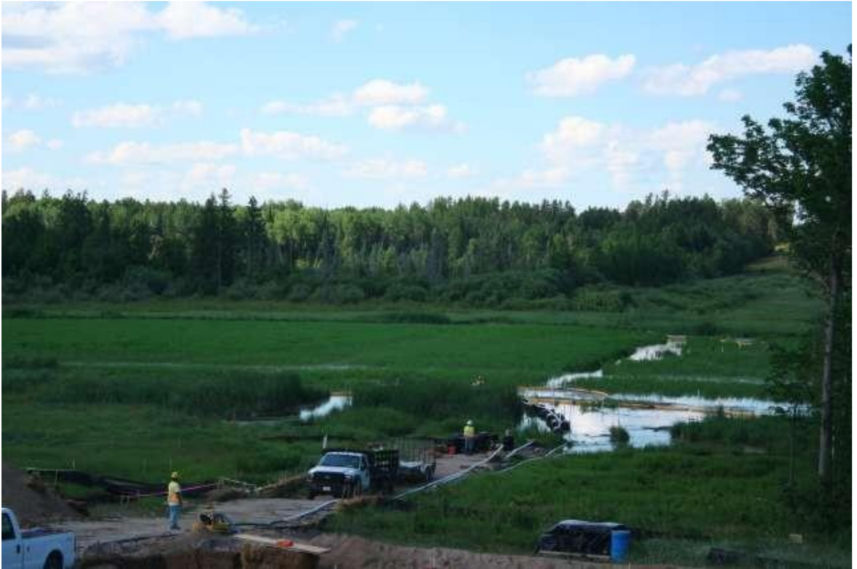
From S, view of Hay Creek clean-up operation.
