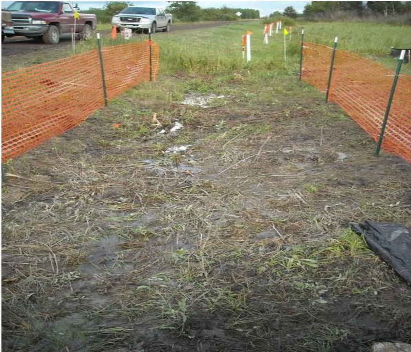
MP 845.80, Frac-out cleanup, W-845D, view east.
