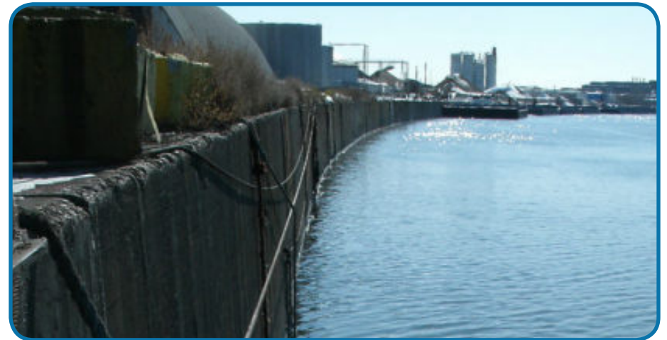
Dock Wall at the Southport Terminal, Credit: Krech Ojard Associates
