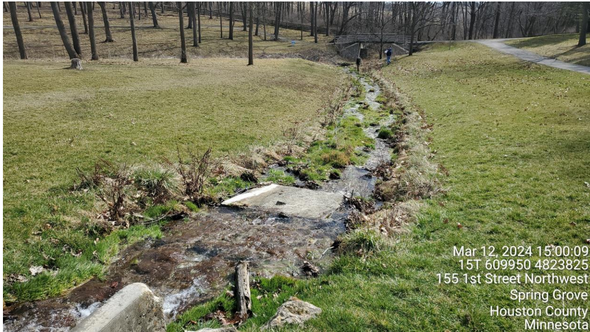
PHOTO NO. 1: View from storm sewer outfall (SW-3) facing south during cascade channel construction in 2020. The surface water (un-named stream) is beyond the far end of the flexamat-lined flow channel, past the trees and upstream of the bridge in the background.
