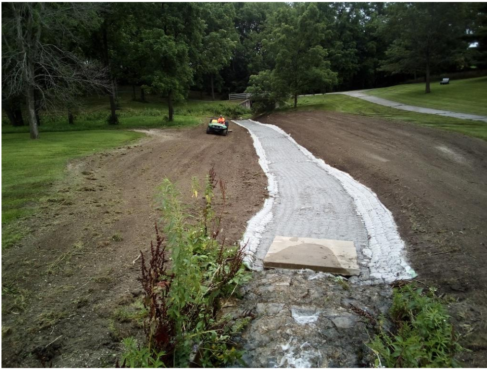
PHOTO NO. 1: View from storm sewer outfall (SW-3) facing south during cascade channel construction in 2020. The surface water (un-named stream) is beyond the far end of the flexamat-lined flow channel, past the trees and upstream of the bridge in the background.
