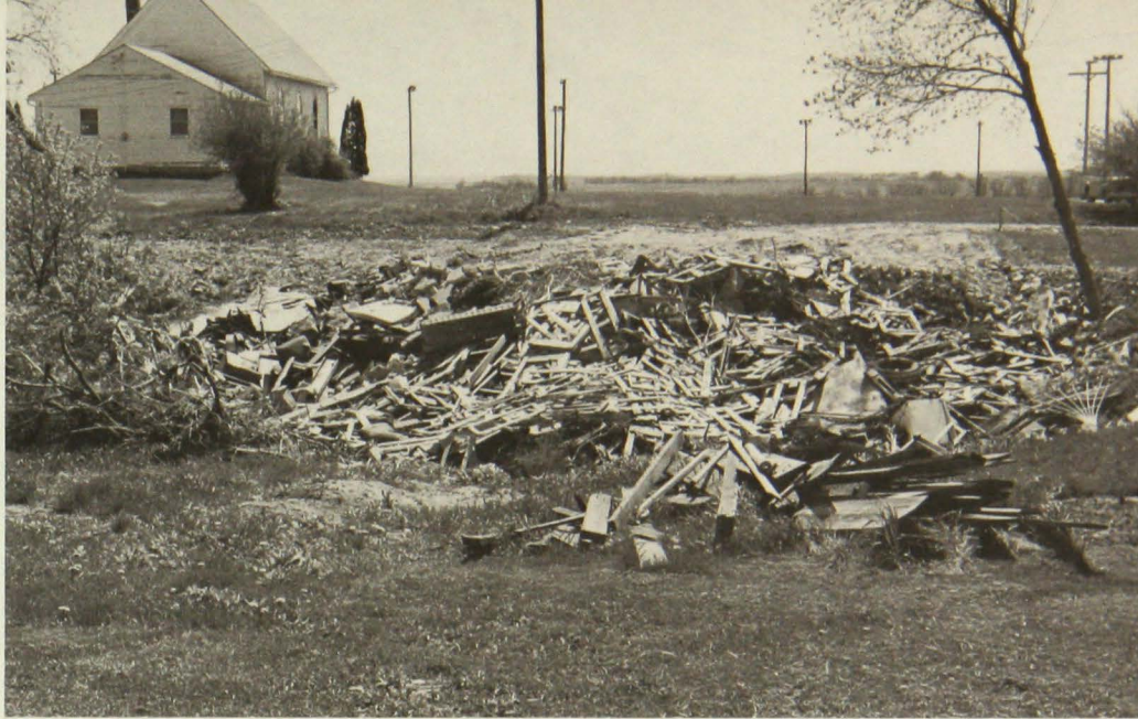
Figure 7. Refuse-filled sinkhole in southeast Minnesota.
