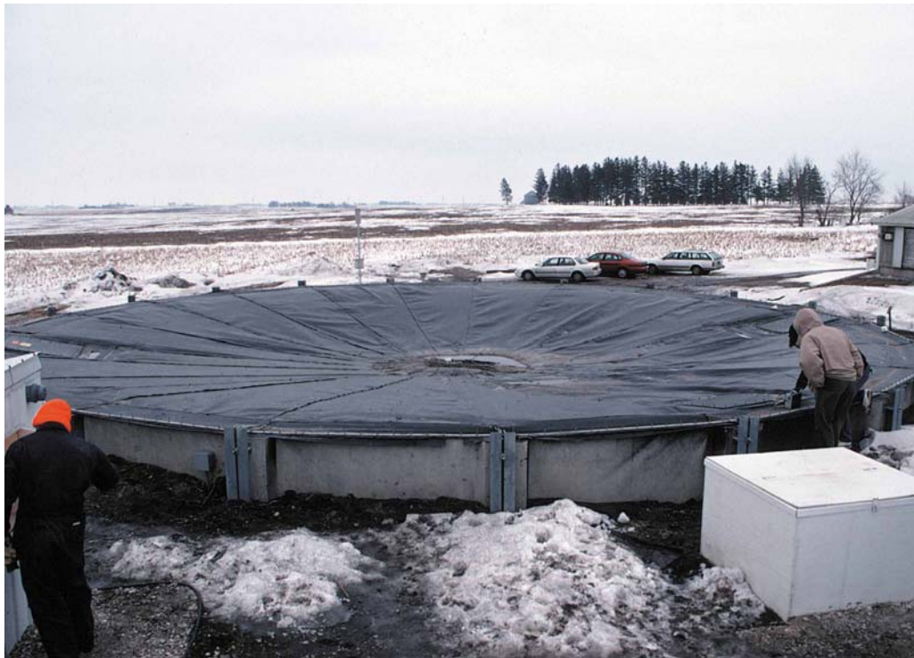
Figure 7.6. Covered manure tank generating methane in Iowa.
