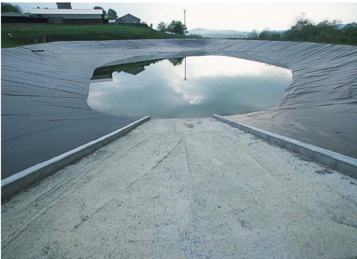
Figure 5.5. A new lagoon with a synthetic geotextile liner to prevent seepage into groundwater.
