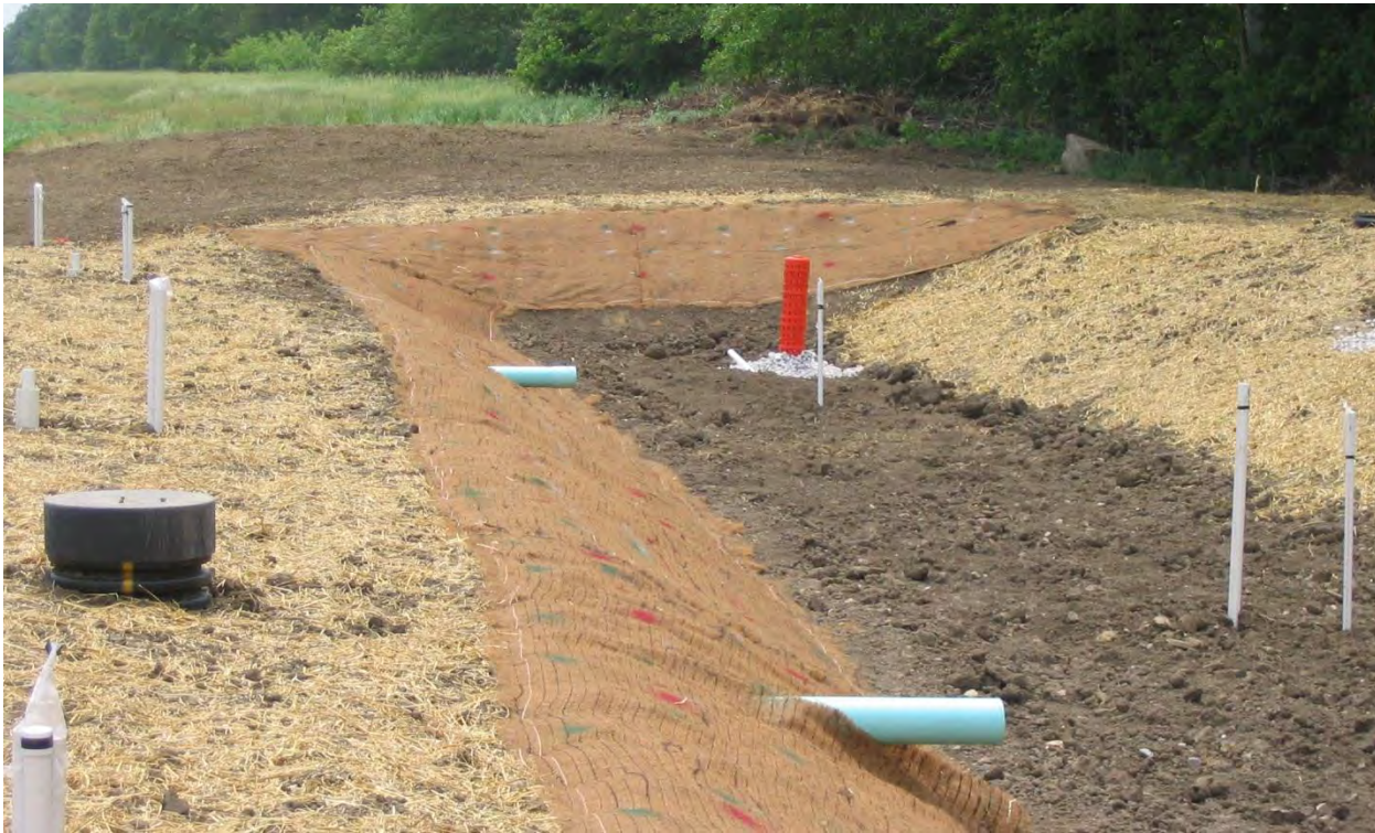
Treatment Wetland under Construction
