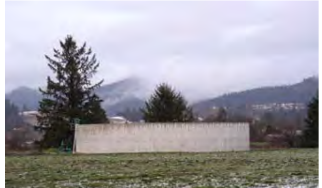
Figure 10D-4 Aboveground storage tank for animal waste ( Photo credit Mitch Cummings, Oregon NRCS )
