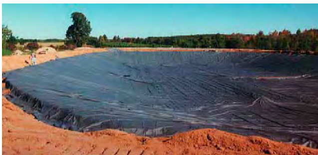
Figure 10D–6 Agricultural waste storage impoundment lined with a geomembrane ( Photo credit NRCS )
