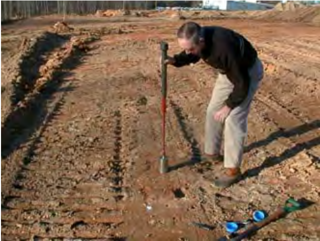
Figure 10D–33 Obtaining undisturbed sample of compacted clay liner using thin-walled drive cylinder
