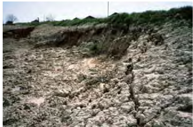
Figure 10D–24 Failure of compacted liner from uplift forces below clay blanket ( Photo credits NRCS, TX )
