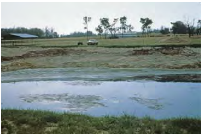
Figure 10D–24 Failure of compacted liner from uplift forces below clay blanket ( Photo credits NRCS, TX )
