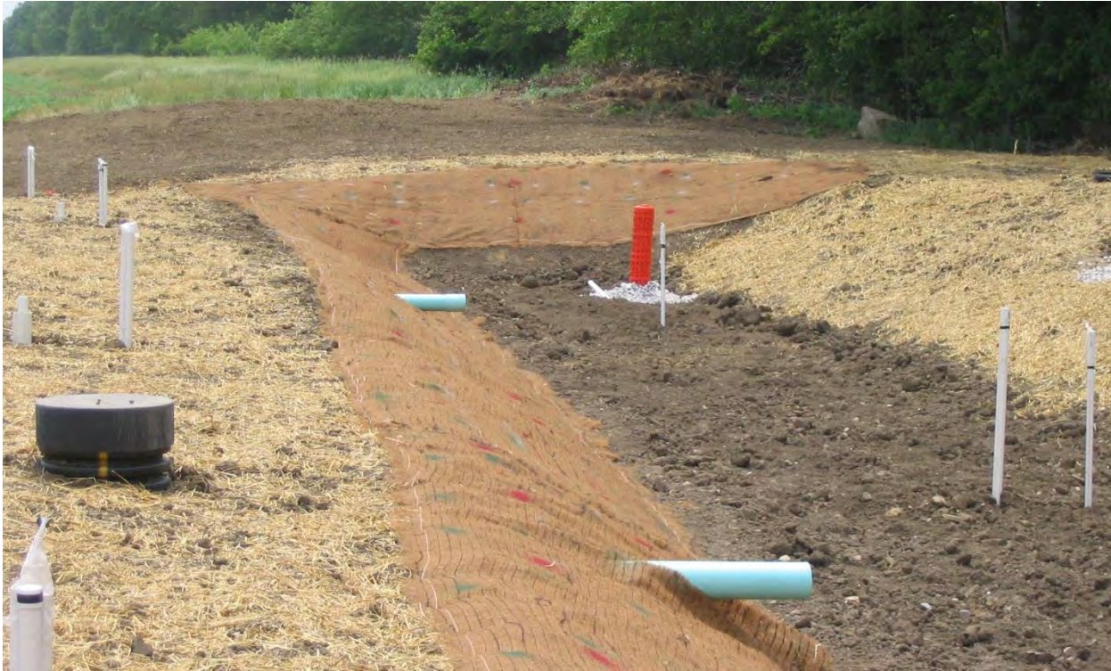
Treatment Wetland under Construction
