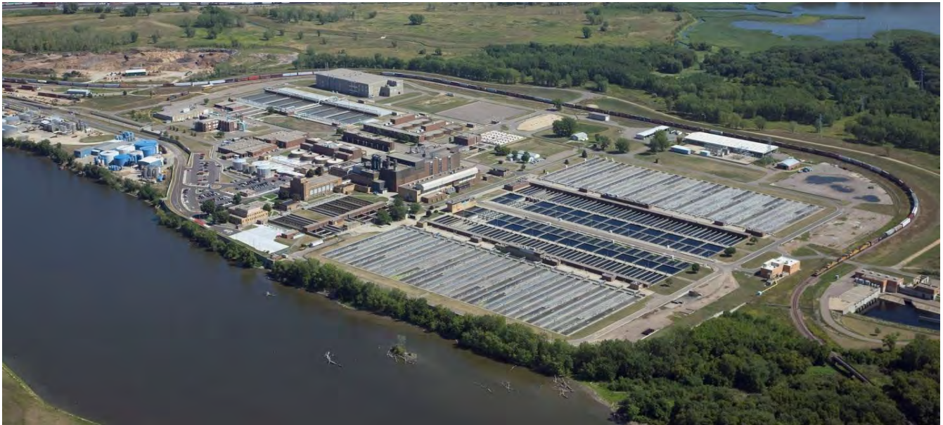
Metropolitan Wastewater Treatment Plant
