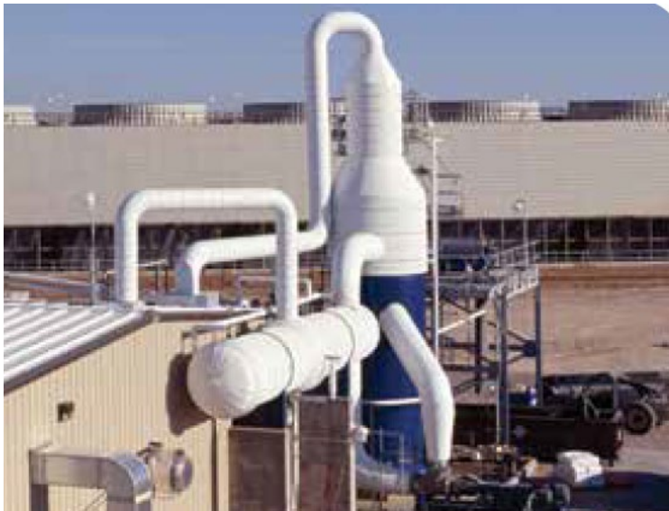
Figure 6 MBD™ Modular Brine Crystallization System – Model 300 (courtesy of Veolia)
