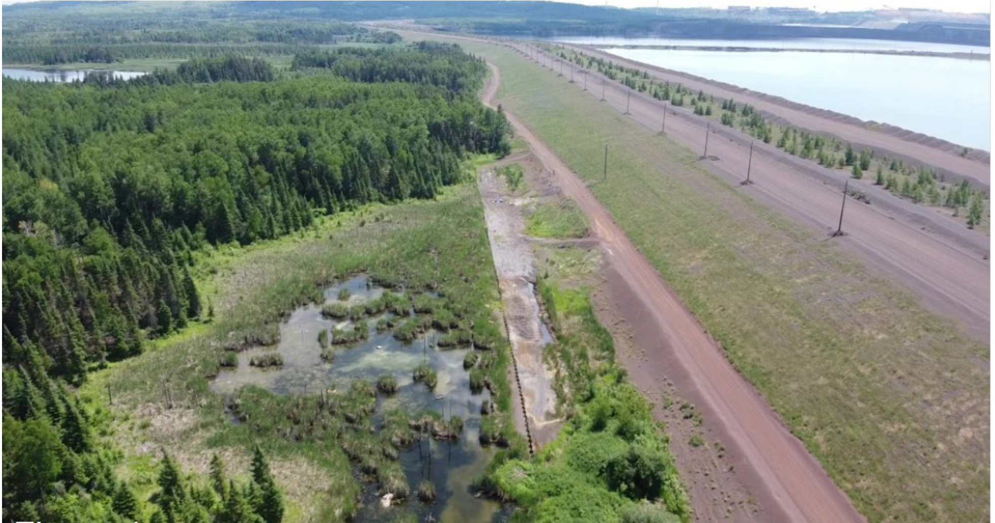
Figure 10. Image of Tailings Basin Perimeter Dike.
