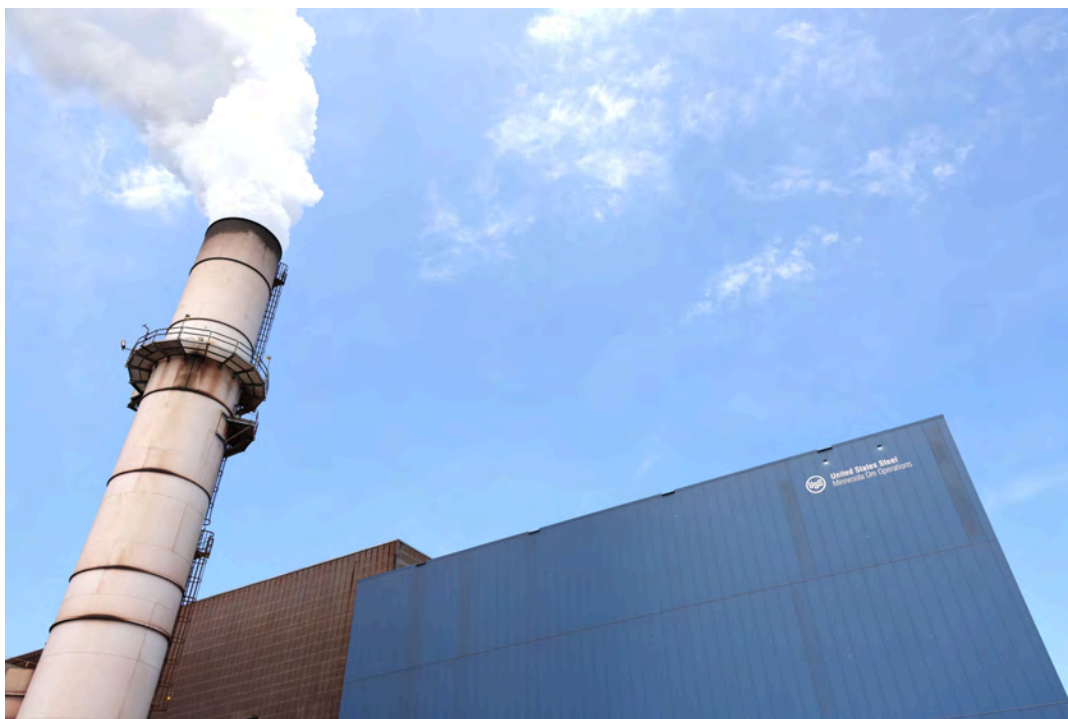
Steam rises from the new Keetac DR-grade pellet plant. Wyatt Buckner / Duluth Media Group
