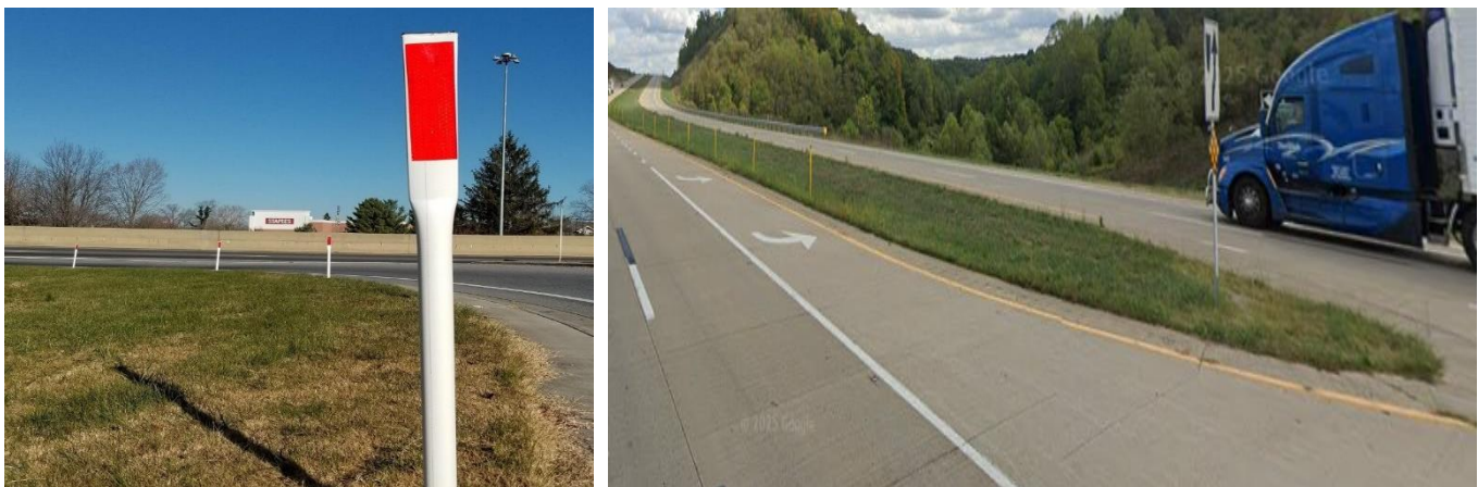
Exhibit 4-1. Post Mounted Delineator (Source: Google)
