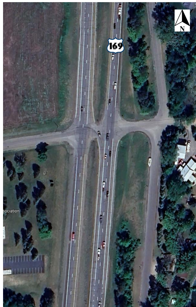
Exhibit 3-12. Location 11: Intersection and Crossover at 273rd Ave
