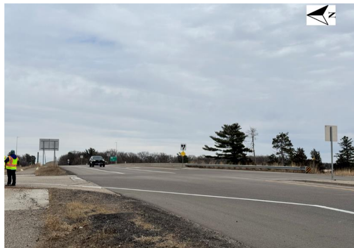
Exhibit 3-15. Location 14: Intersections at West Ramps of US 169 to 289th Ave NW (CSAH 9)
