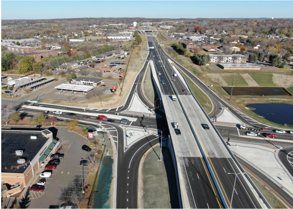
Exhibit 2-14. Elk River Interchange Project (Source: MnDOT)
